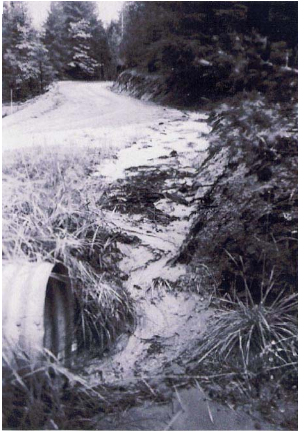
A. Before – Insloped, unsurfaced road on decomposed granitic soils with heavy sediment runoff
