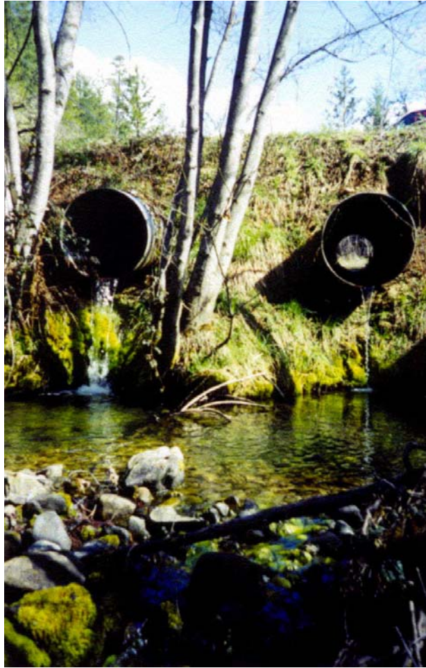
Culverts needing replacement to provide fish passage
