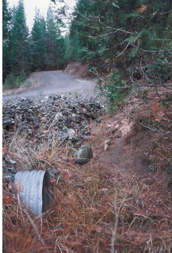
B. After – Outsloped, rocked road with no sediment runoff to culvert and into stream
