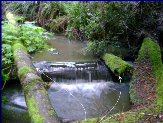
Training logs along bank confine flow
