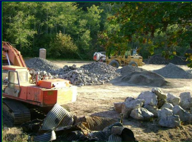
4. Stockpile Engineered Streambed Material onsite. Within a small section of channel, place material in correct proportions and mix with excavator bucket ...
