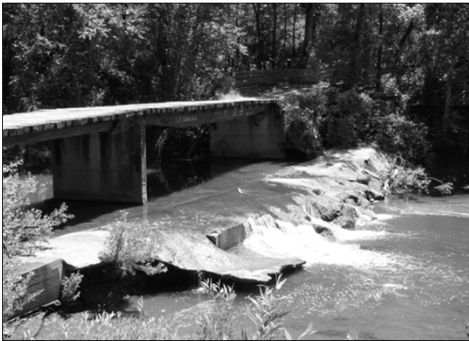
Perched Outlet – Water Line Encasement
