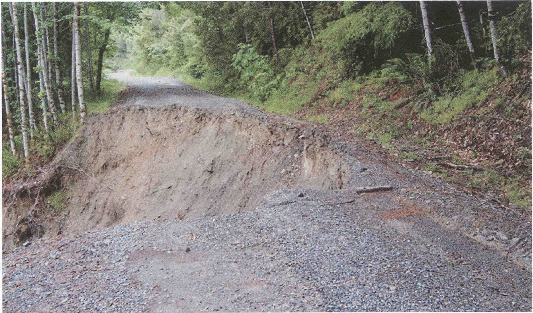
Road failure caused by stream undercutting
