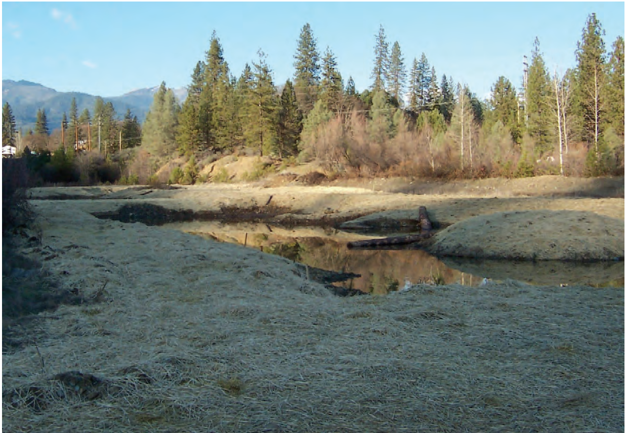
Upper Photo: Upper middle pond after wetlands construction. The island, woody debris, and irregular pond edges are visible. Seedling and other vegetation efforts were planned based on anticipated water levels that were monitored prior to construction and during the first post project winter storms. The areas were seeded and mulched.
