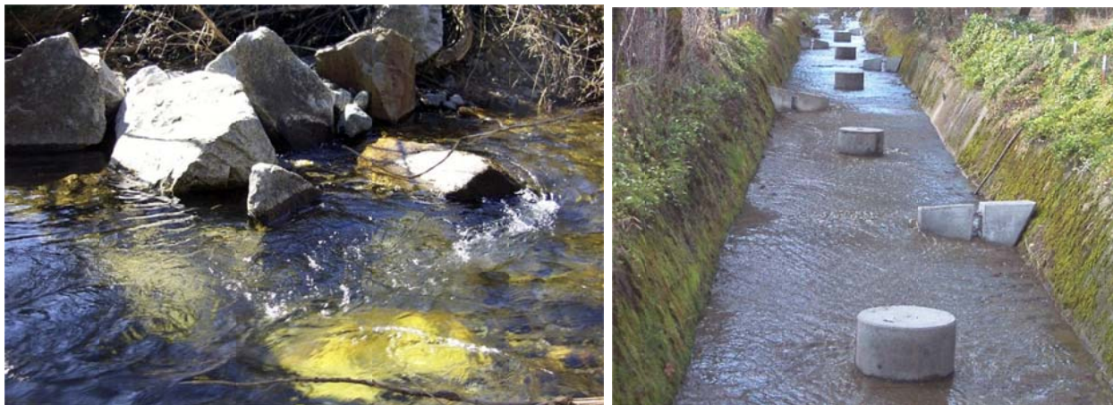
Photo 7 (left): Boulder cluster in Lee Fong Park constructed in 19991 as part of Trinity County's Urban Stream Project (photo taken in 2006). Photo 8 (right): Resting structures within the Forest Service compound.
