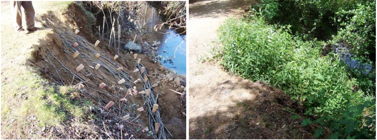
Photos 9 and 10: A stream bank undercut in the January 2006 storms had been proposed to be rip-rapped, but willow mattress bio-engineering techniques were used instead.
