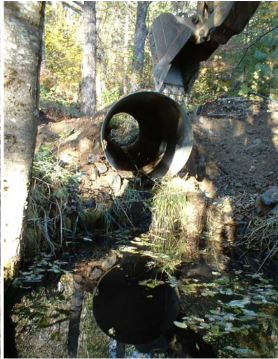
Photo Series 2 (Pictures 1-6): Before and during construction of Finley Crossing including before( upper left); excavating out the 42" CMP (upper middle and right); preparing the bed for the new CMP (lower left) and placing the first segment and band (Lower middle and right). All photos taken October 27, 2009)
