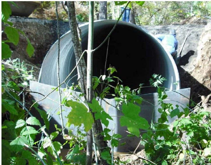
Photo Series 8: View of outlet: Before and during showing upstream channel & culvert and plate in place but no flow or rock slope protection in place. Lower Right is following winter storm flows of January & early February 2010
