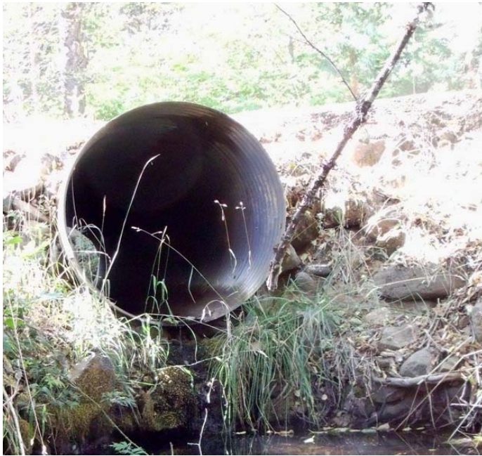
Photo Series 8: View of outlet: Before and during showing upstream channel & culvert and plate in place but no flow or rock slope protection in place. Lower Right is following winter storm flows of January & early February 2010
