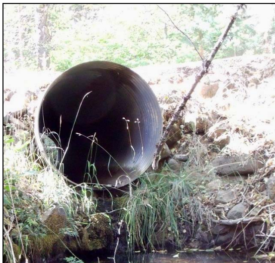
Pre-project photo of perched 42-inch culvert
