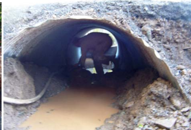
Photo Series 5: Installing streambed Mix: Upper left- CMP w/plate ready to install; Upper middle- the inlet is filled with mix. Upper right- inlet mix beginning to be fed into CMP. Middle left and center photos- feeding streambed mix into culvert. Middle right photo- ramp to feed mix into outlet end of CMP. Lower left and right photos- distributing mix. Lower middle- pressure washing mix in culvert.
