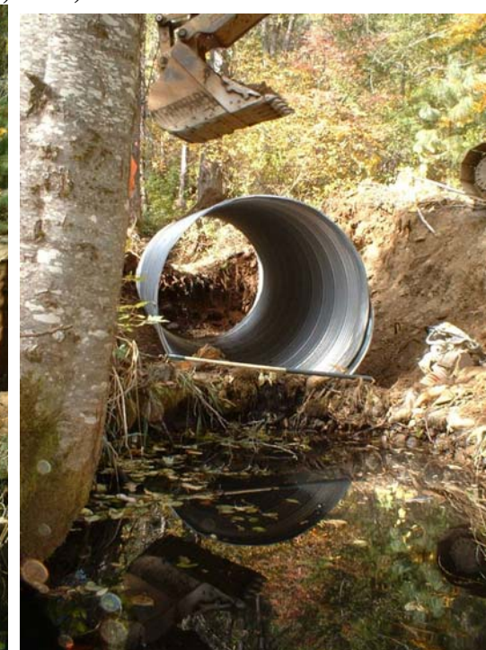
Photo Series 2 (Pictures 1-6): Before and during construction of Finley Crossing including before( upper left); excavating out the 42" CMP (upper middle and right); preparing the bed for the new CMP (lower left) and placing the first segment and band (Lower middle and right). All photos taken October 27, 2009)
