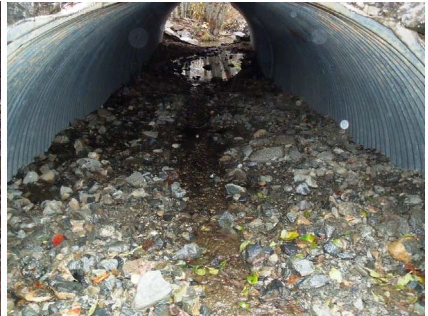
Photo Series 6: Placing streambed mix (Upper left). Mix immediately after completion of jetting on November 3 rd , 2009 (upper right). Mix after first high flows February 3 rd , 2010 (lower)
