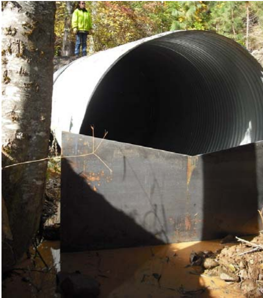
Photo Series 2 (Pictures 7-9): Left: Outlet showing the steel plate during jetting and placement of bedload material (November 1, 2009). Middle: Outlet after bedload material has been placed and jetted and rock slope boulder placed (November 3, 2009). Right: Outlet flow during the receding end of a winter storm (February 2, 2010)
