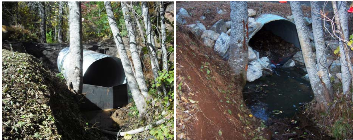
Photo Series 4: Water Quality Monitoring: There was minimal surface water flow during the project. Surface flow was routed around the site in a 2" HDPE pipe. Upper left Photo the outlet pool was protected during construction by retaining a 4' wide portion of the pre-project perched streambed forming a barrier between the work area and any water (not the pool in the lower 1/3 of the photo). Upper middle and right photos and lower left photo- during jetting of streambed material all water was pumped out of the pool. Lower right photo- Once jetting was completed the pool was washed with a low pressure hose to remove all sediment before flow was routed back into stream.
