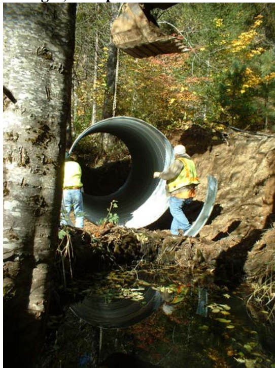
Photo Series 2 (Pictures 1-6): Before and during construction of Finley Crossing including before( upper left); excavating out the 42" CMP (upper middle and right); preparing the bed for the new CMP (lower left) and placing the first segment and band (Lower middle and right). All photos taken October 27, 2009)
