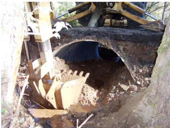
Photo Series 5: Installing streambed Mix: Upper left- CMP w/plate ready to install; Upper middle- the inlet is filled with mix. Upper right- inlet mix beginning to be fed into CMP. Middle left and center photos- feeding streambed mix into culvert. Middle right photo- ramp to feed mix into outlet end of CMP. Lower left and right photos- distributing mix. Lower middle- pressure washing mix in culvert.
