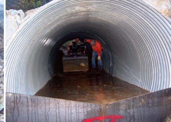
Photo Series 5: Installing streambed Mix: Upper left- CMP w/plate ready to install; Upper middle- the inlet is filled with mix. Upper right- inlet mix beginning to be fed into CMP. Middle left and center photos- feeding streambed mix into culvert. Middle right photo- ramp to feed mix into outlet end of CMP. Lower left and right photos- distributing mix. Lower middle- pressure washing mix in culvert.
