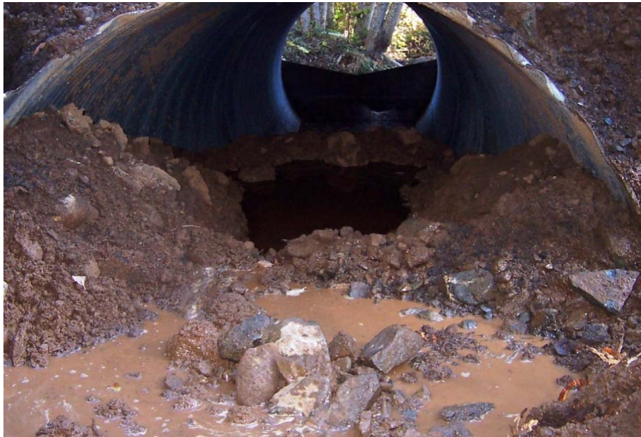
Photo Series 6: Placing streambed mix (Upper left). Mix immediately after completion of jetting on November 3 rd , 2009 (upper right). Mix after first high flows February 3 rd , 2010 (lower)
