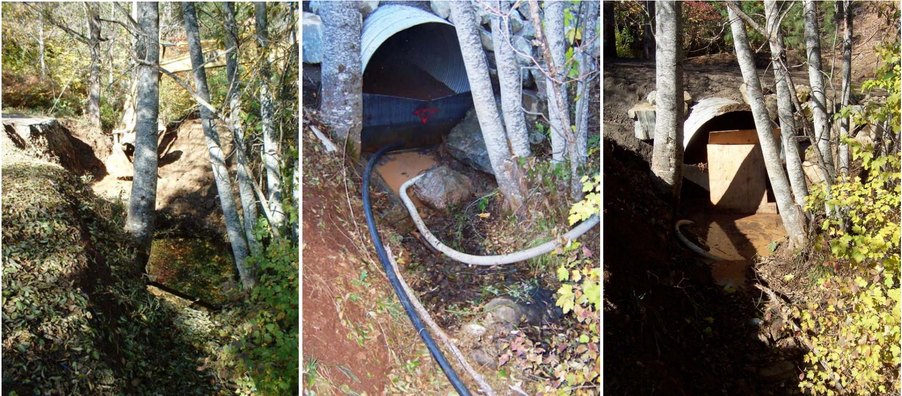
Photo Series 4: Water Quality Monitoring: There was minimal surface water flow during the project. Surface flow was routed around the site in a 2" HDPE pipe. Upper left Photo the outlet pool was protected during construction by retaining a 4' wide portion of the pre-project perched streambed forming a barrier between the work area and any water (not the pool in the lower 1/3 of the photo). Upper middle and right photos and lower left photo- during jetting of streambed material all water was pumped out of the pool. Lower right photo- Once jetting was completed the pool was washed with a low pressure hose to remove all sediment before flow was routed back into stream.
