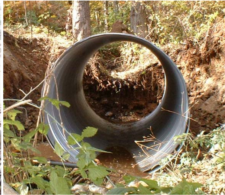
Photo Series 8: View of outlet: Before and during showing upstream channel & culvert and plate in place but no flow or rock slope protection in place. Lower Right is following winter storm flows of January & early February 2010
