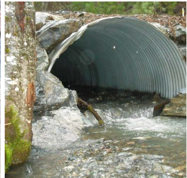
Photo Series 2 (Pictures 7-9): Left: Outlet showing the steel plate during jetting and placement of bedload material (November 1, 2009). Middle: Outlet after bedload material has been placed and jetted and rock slope boulder placed (November 3, 2009). Right: Outlet flow during the receding end of a winter storm (February 2, 2010)
