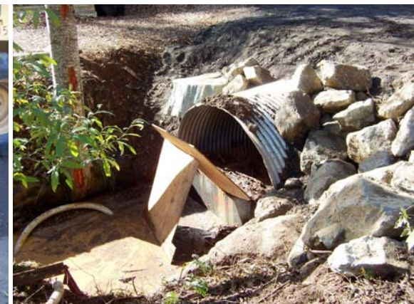
Photo Series 5: Installing streambed Mix: Upper left- CMP w/plate ready to install; Upper middle- the inlet is filled with mix. Upper right- inlet mix beginning to be fed into CMP. Middle left and center photos- feeding streambed mix into culvert. Middle right photo- ramp to feed mix into outlet end of CMP. Lower left and right photos- distributing mix. Lower middle- pressure washing mix in culvert.
