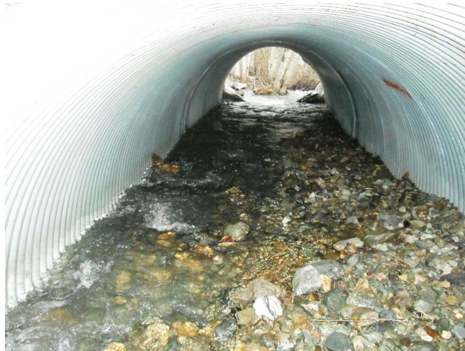
Photo Series 6: Placing streambed mix (Upper left). Mix immediately after completion of jetting on November 3 rd , 2009 (upper right). Mix after first high flows February 3 rd , 2010 (lower)
