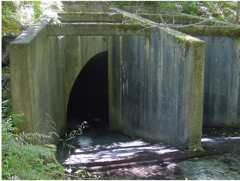
Figure 2. 3. Concrete arch culvert with a concrete inlet apron and debris wall. If the apron has a steeper slope than the culvert, the apron may cause a velocity barrier to fish passage.
