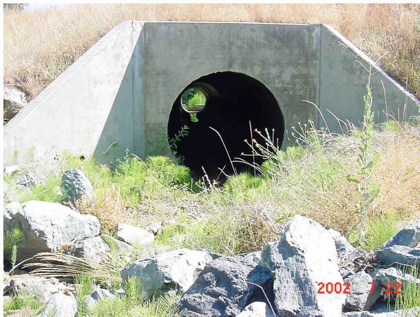
Figure 2.6. Wingwalls and headwalls guide flow into culverts and protect fill slopes from erosion.
