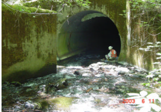
Culvert Inlet and debris blocker
