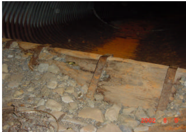
Weirs in Culvert 1
