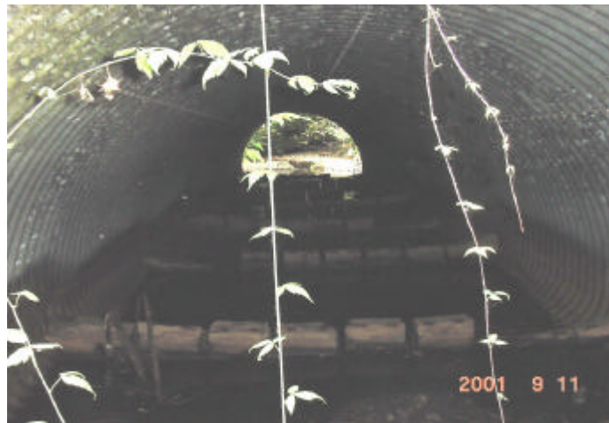
Wooden baffles in culvert
