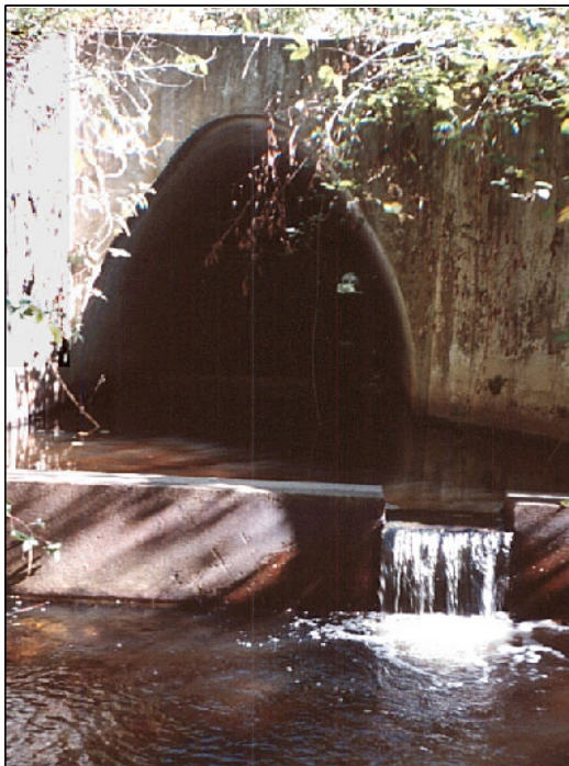
Figure 2.4. The picture on the left shows a concrete outlet weir with a low flow notch. The picture on the right shows multiple boulder weirs installed to mitigate a perched outlet.
