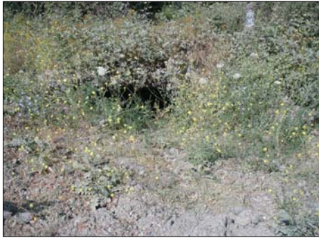
Left: Shows a 6-ft-diameter sinkhole on the road shoulder due to high flows coming up through the failed section of culvert. The sinkhole is located ~ 10 feet from the edge of the slipout (right) .
