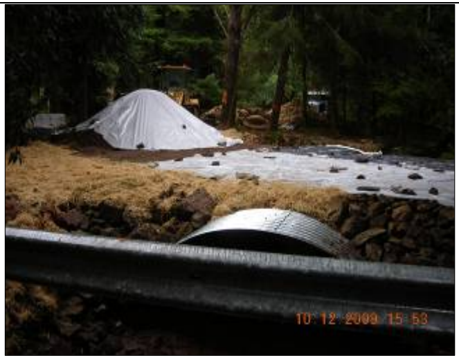
Ancestor Creek Migration Barrier Removal Project- Erosion and Sediment Control BMPs in response to forecast rain.
