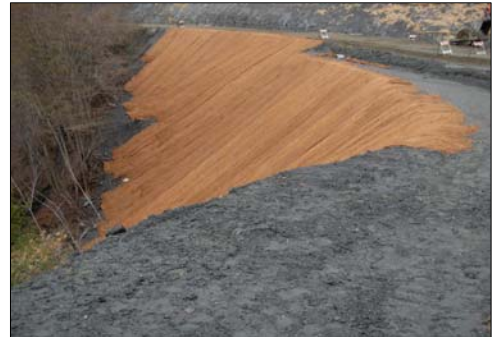
Right: Shows coconut fiber geotextile matting installed on downslope. Upslope side contains straw wattles and mulch.
