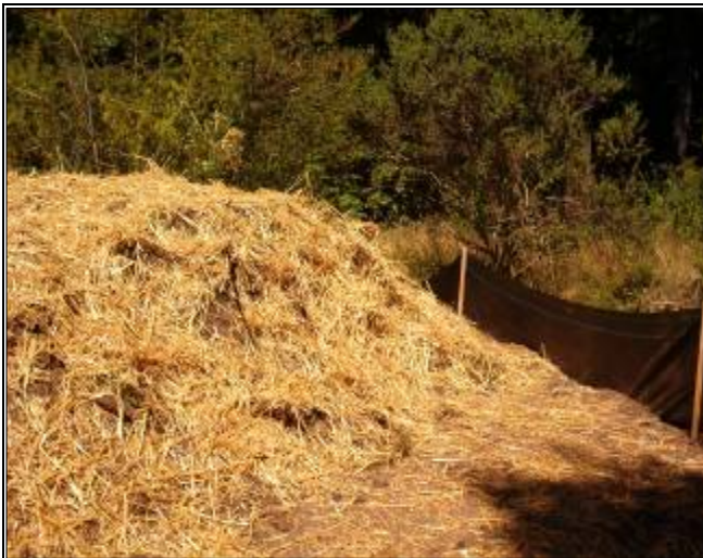
Stockpile - erosion and sediment control BMPs – straw and sediment fence protection from erosion.
