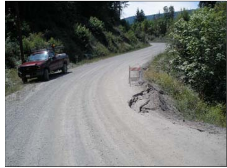
Left: Shows a 6-ft-diameter sinkhole on the road shoulder due to high flows coming up through the failed section of culvert. The sinkhole is located ~ 10 feet from the edge of the slipout (right) .
