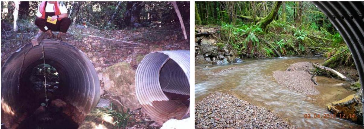
The Ancestor Creek crossing consisted of a 7' and 3' diameter culvert (left). These pipes were replaced with a 16' wide, embedded multiplate arch culvert (above right and below). Installing culverts utilizing the active channel design can allow for natural stream function and large wood placement, as depicted below.
