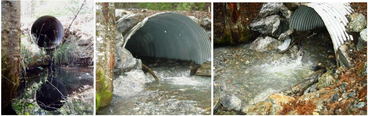
Above Left: Finley Gulch was a 42" diameter culvert with a 2' jump at the outlet. It was replaced with an 84" embedded culvert (center and right photos) and designed with a 5" jump into the outlet.
