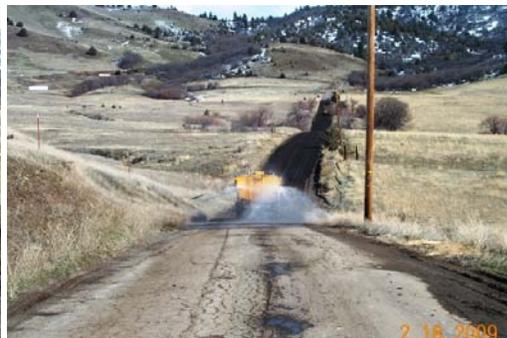
All five counties use asphalt grindings to surface unpaved roads or resurface chip-sealed roads. The photos above demonstrate placement of grindings on York Road (Siskiyou County).
