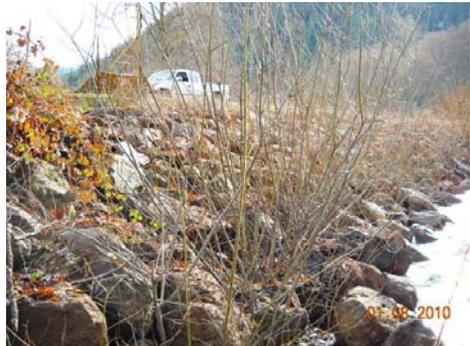
Above: Bar Road Storm Repair (Siskiyou County) repairs made in 2008 (after the 2006 storm damage) included implementing joint planting within rock slope protection. Photos taken January 2010.
