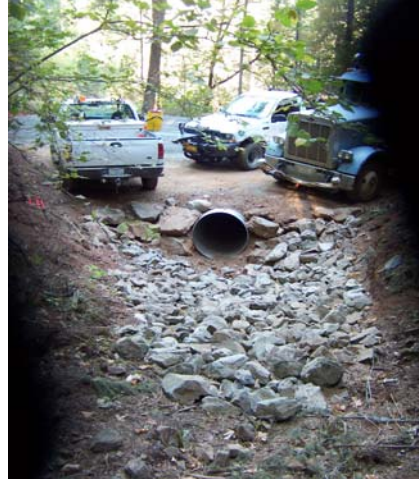
Same Site with 48" culvert installed & critical dip (below) – Sept 2008
