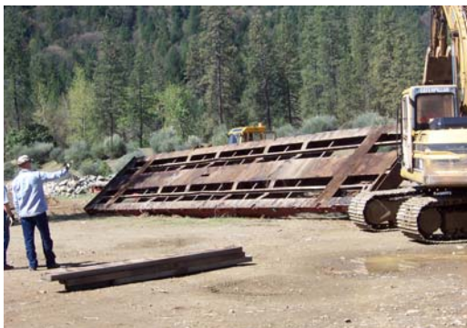
Loading the 55' railcar bridge from the Trinity County yard for transport to the Siskiyou County yard for painting & upgrading
