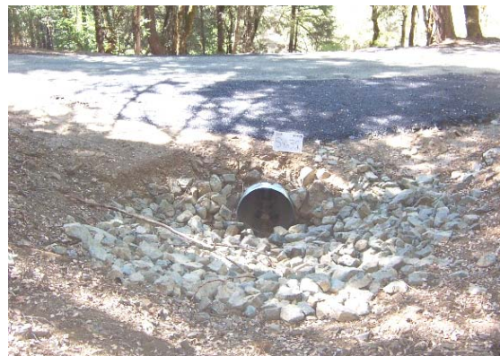
New culvert with armored inlet & outlet
