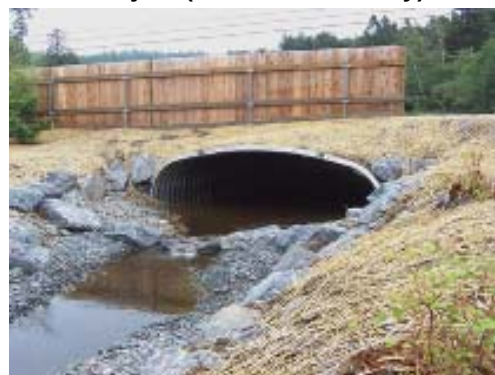
Bottomless arch installed in 2007
