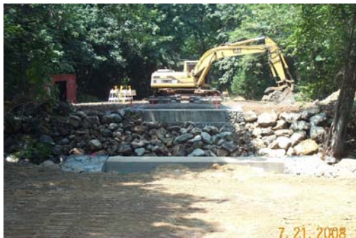
Construction of gabion abutment
