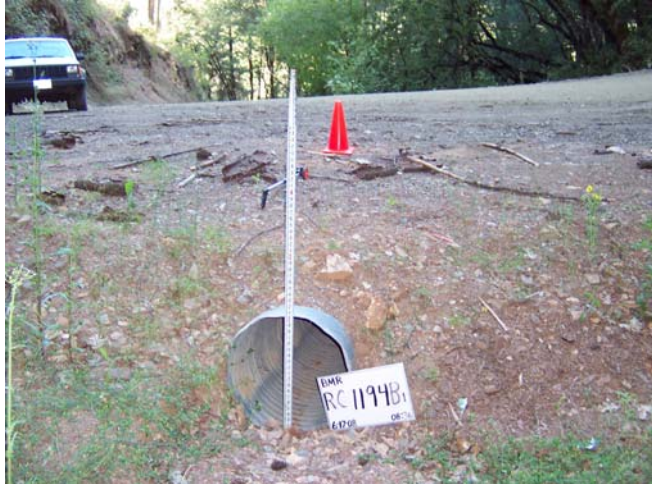
24" stream crossing culvert inlet on Browns Mountain Road prior to upgrade – June 2008
