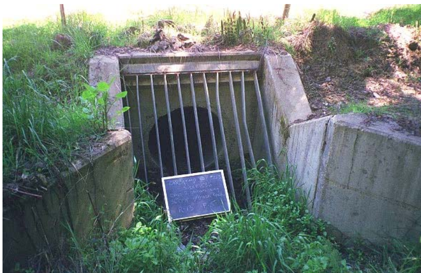
Class II stream crossing with a nicely installed inlet, not a fish-bearing stream Orr Springs Road, Mendocino County
