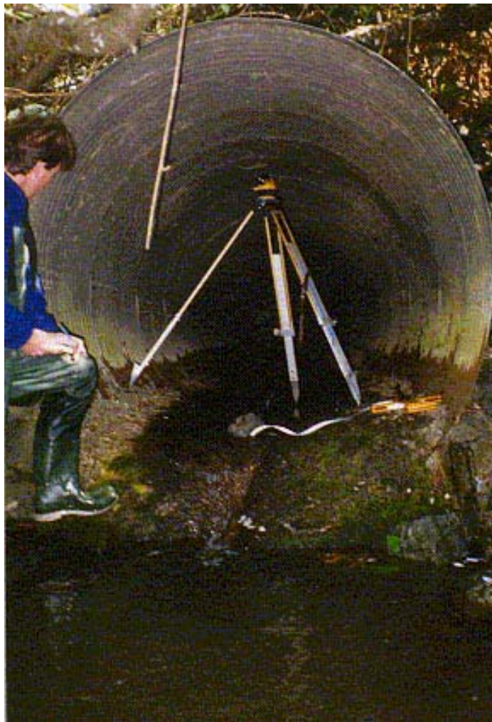
Measuring an existing culvert for size and slope
