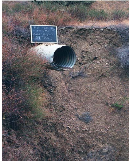
Shotgun outlet causing erosion and sediment delivery to stream
