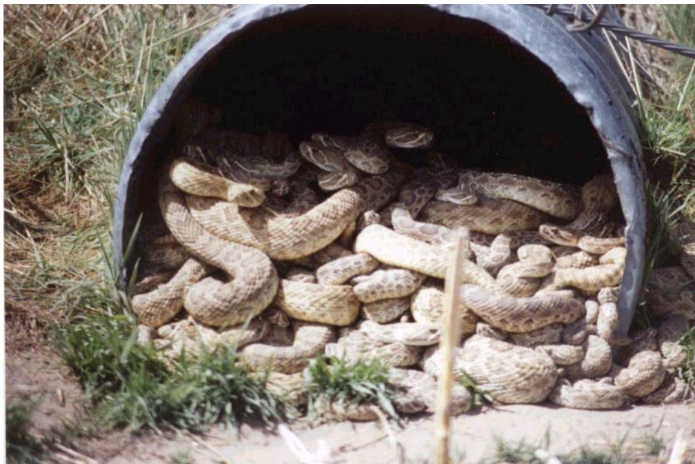
A culvert that needs cleaning. See also: Hazardous Materials Photo source: Caltrans, Tehama County, CA (2002)
