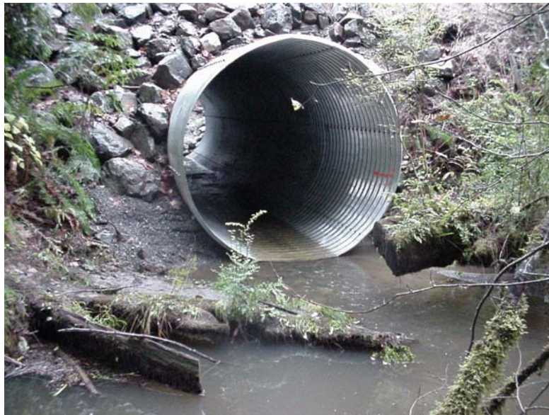
A successful culvert replacement (Morrison Gulch, Humboldt County)
