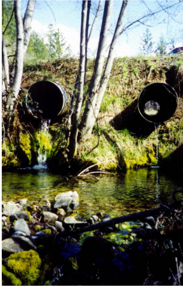
Culverts needing replacement to provide fish passage
