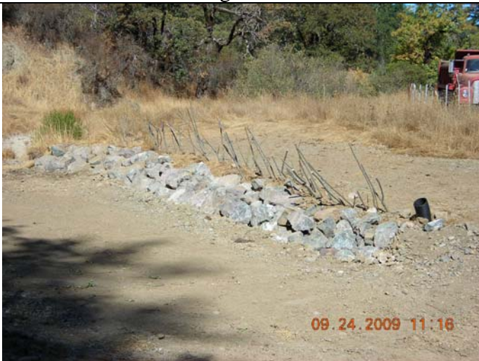
Down stream- live willow staking with subsurface perforated pipe for irrigation.
