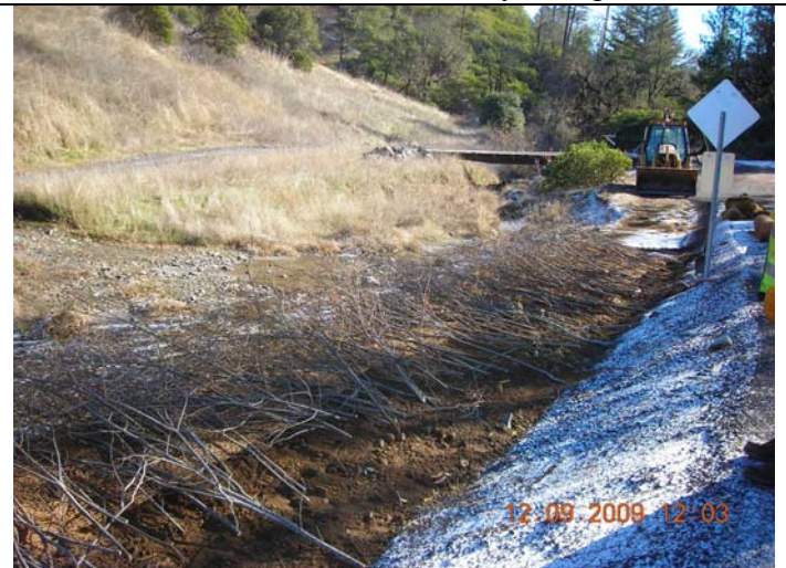
Up stream- brush layering in progress.
