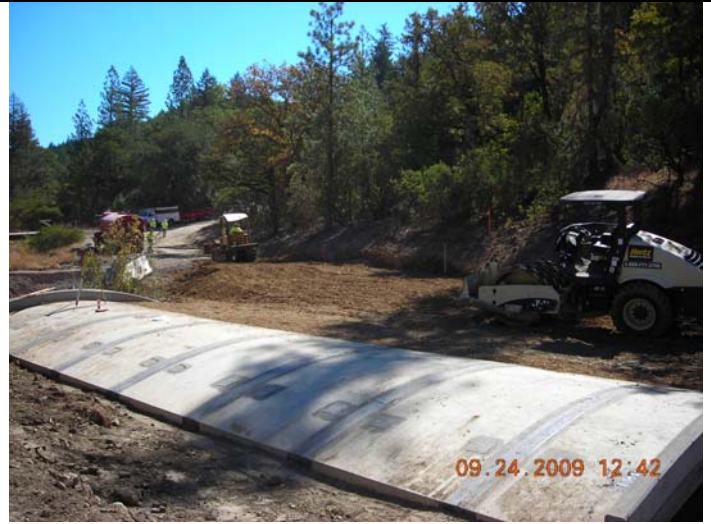
Structure backfill and roadway realignment.
