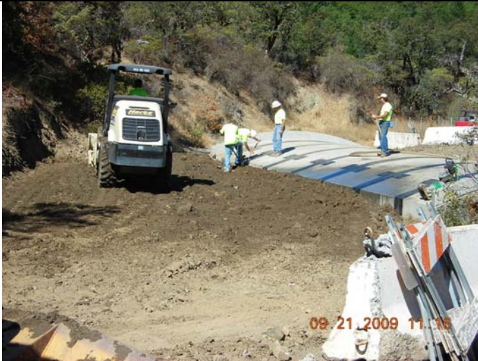
Backfilling the structure.
