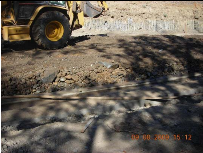
Select streambed strata placement, fines portion prior to jetting in.
