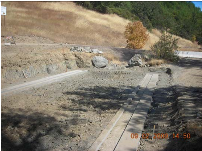
Strip footings are in and getting ready to place select streambed strata mix.
