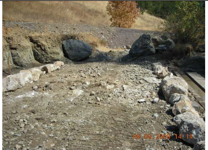
Final streambed strata prior to establishment of low flow channel.
