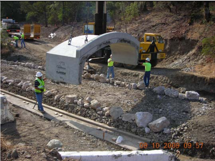
Placing the first concrete arch element.
