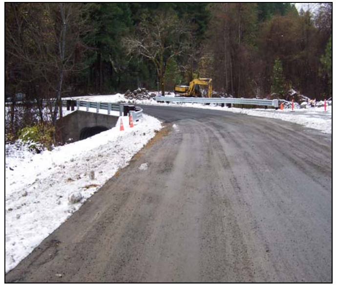
Roadway surfaces and guardrails installed at Crossing #1 (left ) and Crossing #2 (right)
