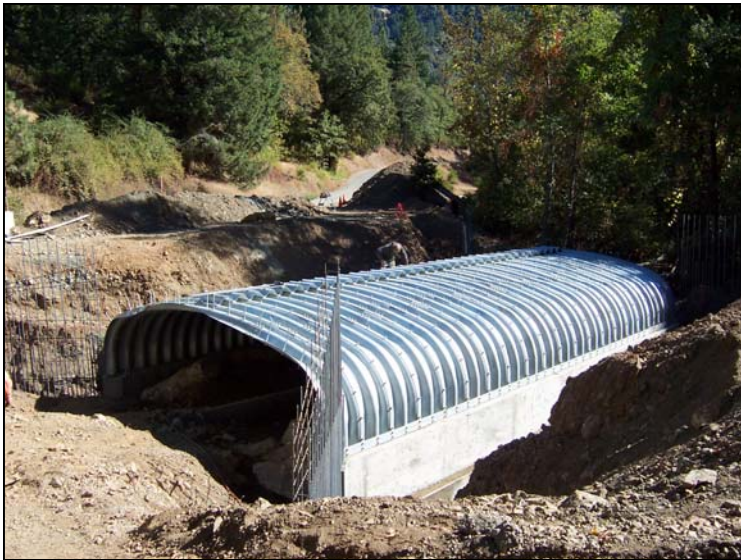
The concrete footings on Crossing #2 were set below ground level and backfilled. Shorter stemwalls (right) are exposed and the arch is attached to the stemwall surface
