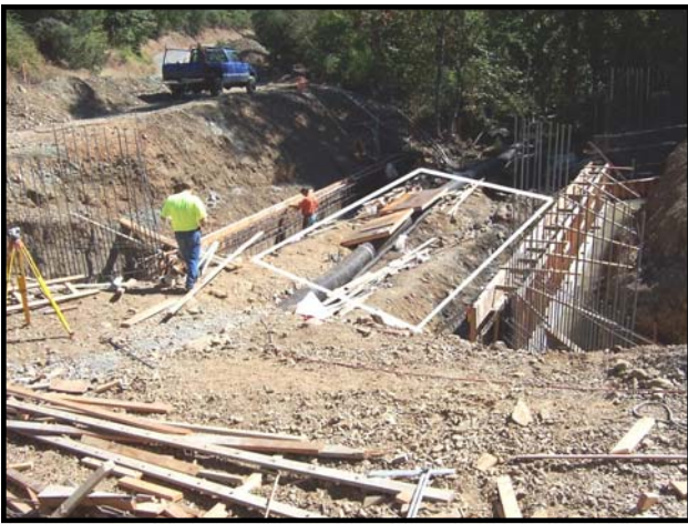
The concrete footings on Crossing #2 were set below ground level and backfilled. Shorter stemwalls (right) are exposed and the arch is attached to the stemwall surface
