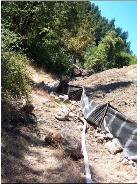
Top & Left— Silt fencing on fill material to be re-used as structural backfill on the arches
