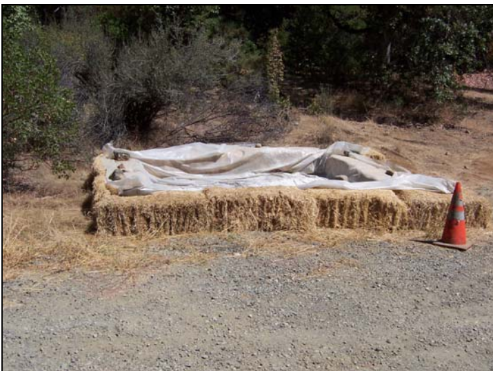
Bottom— Straw bale concrete wash stations for tools and concrete pump trucks
