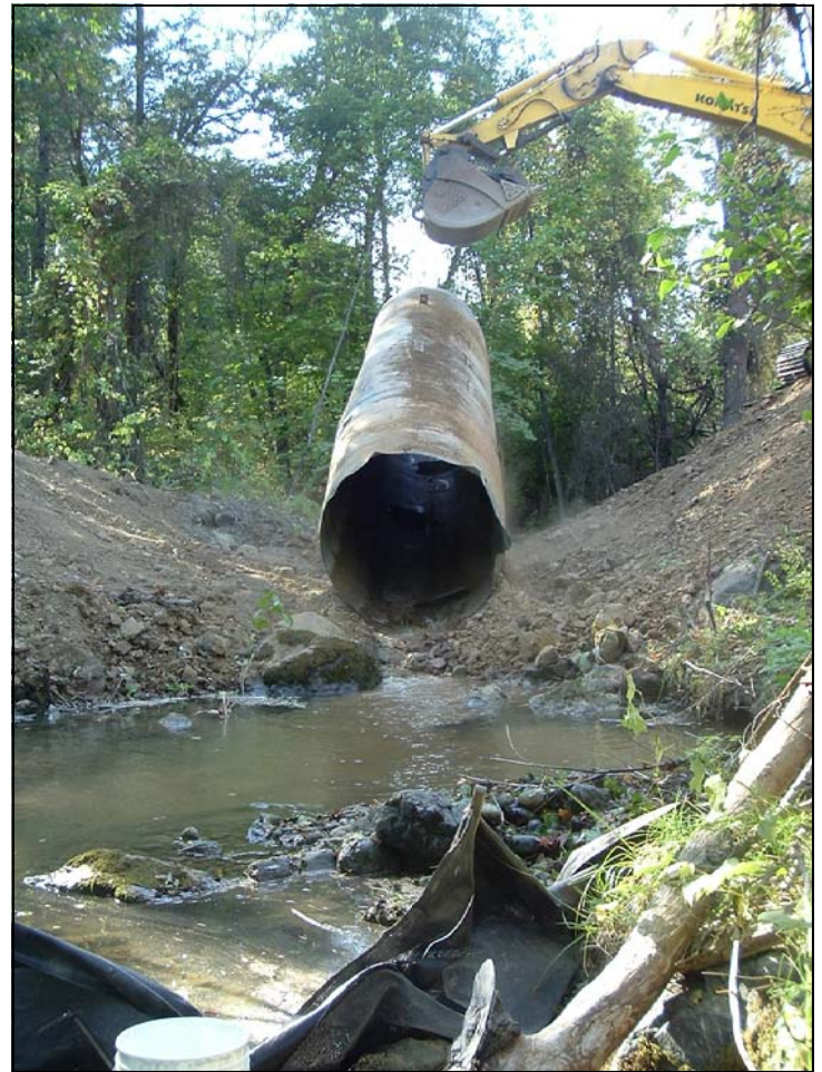
Above —Removing the culvert
