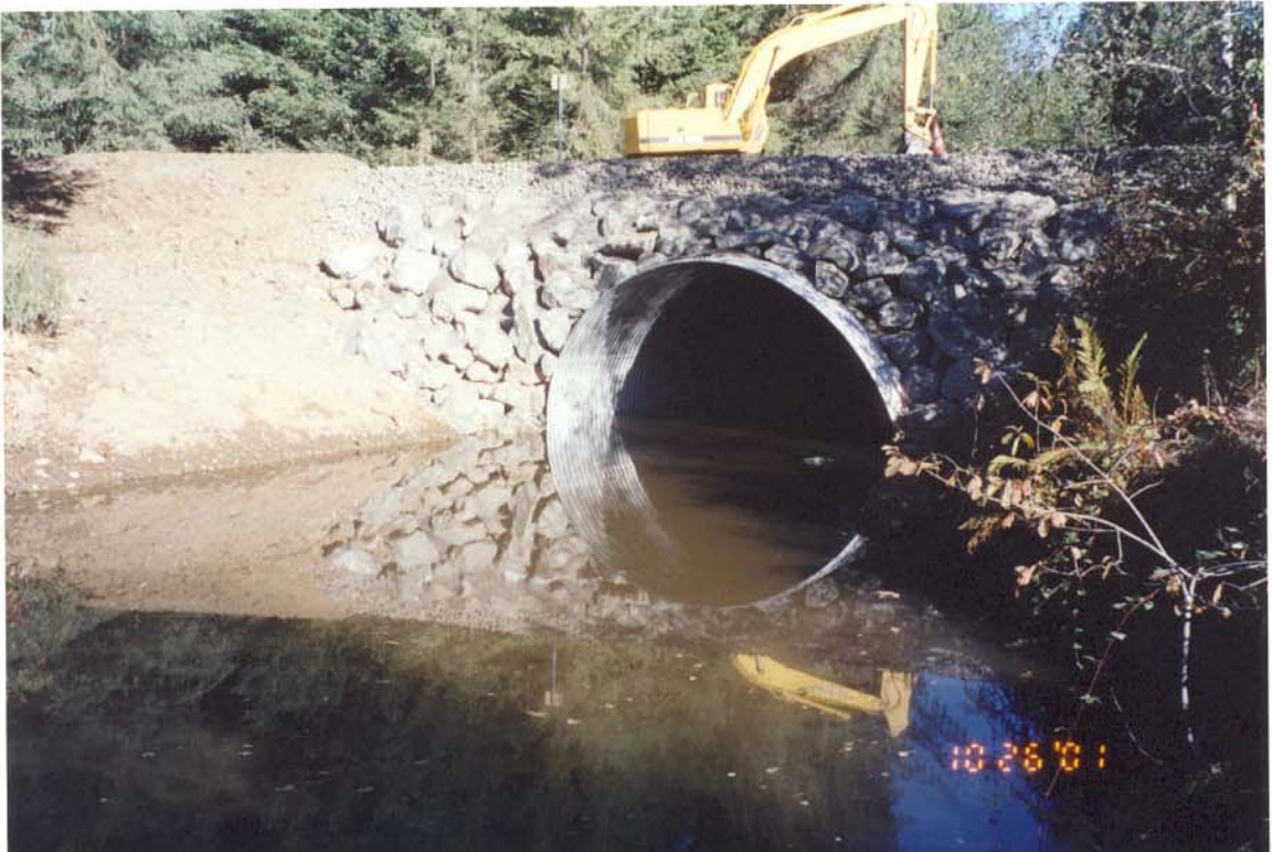
Outlet Rip Rap before Being Concreted
