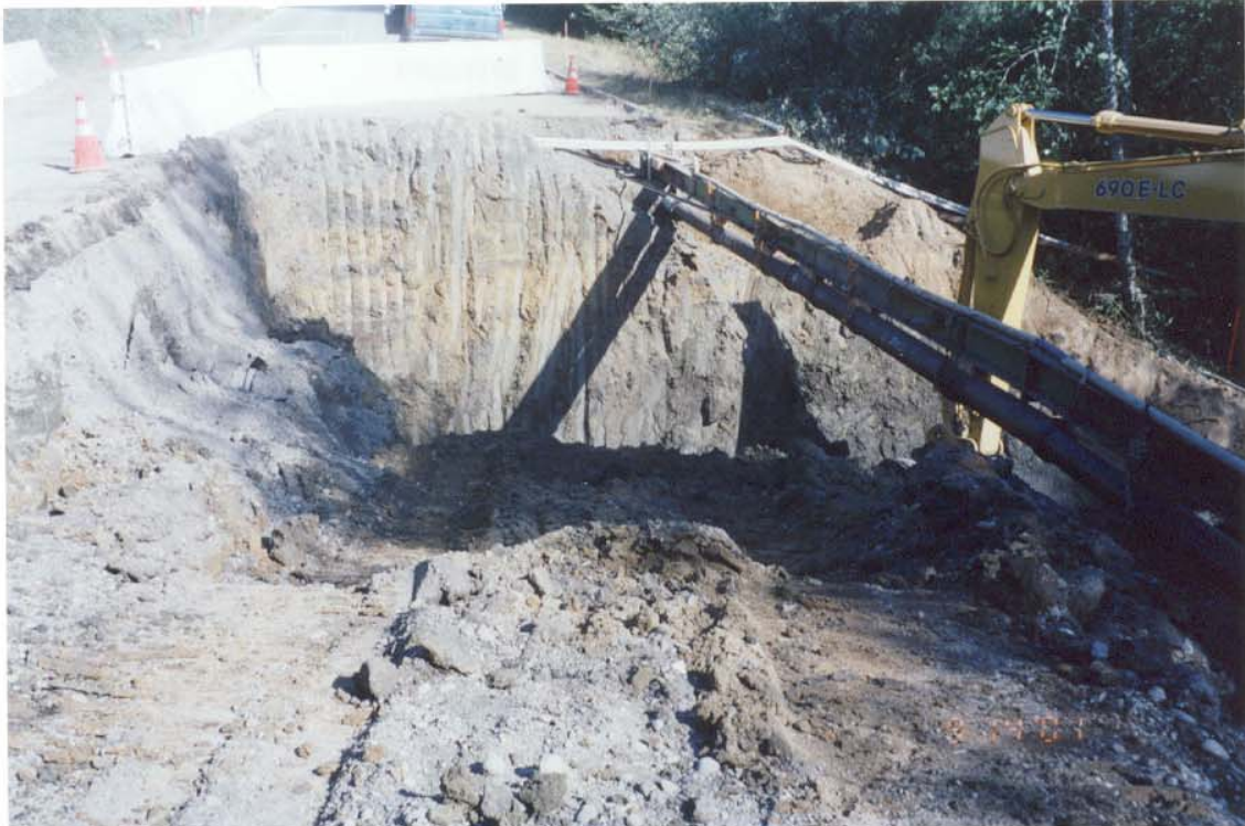
Waterline Suspended above Excavation
