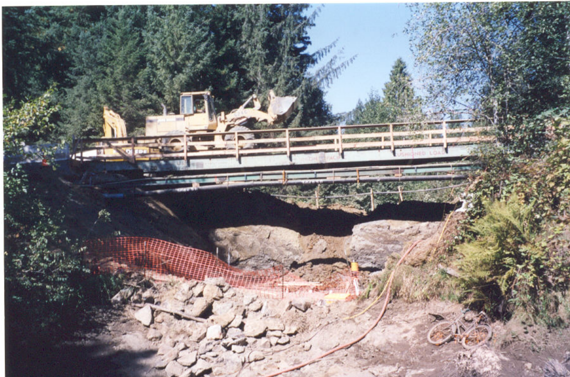
Temporary Flatcar Bridge Viewed from Downstream
