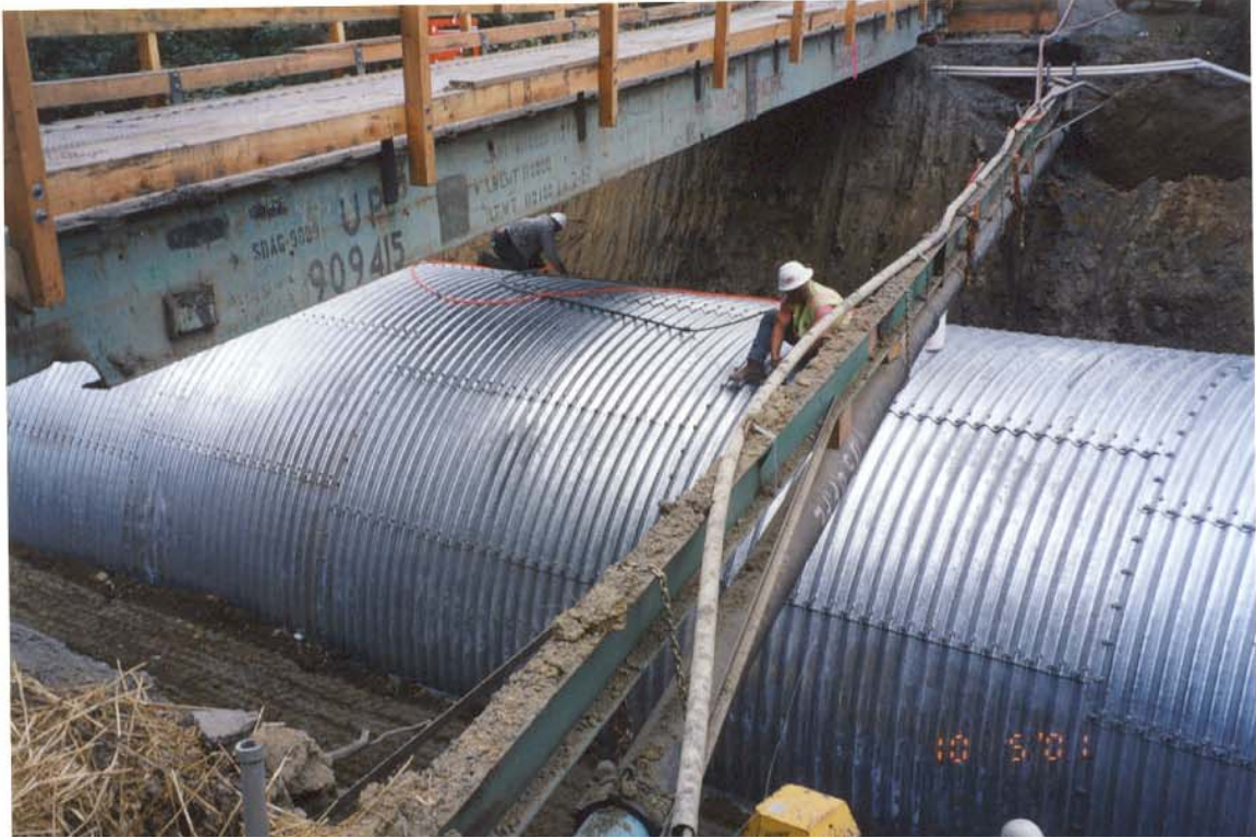
Bolt Tightening and Backfill
