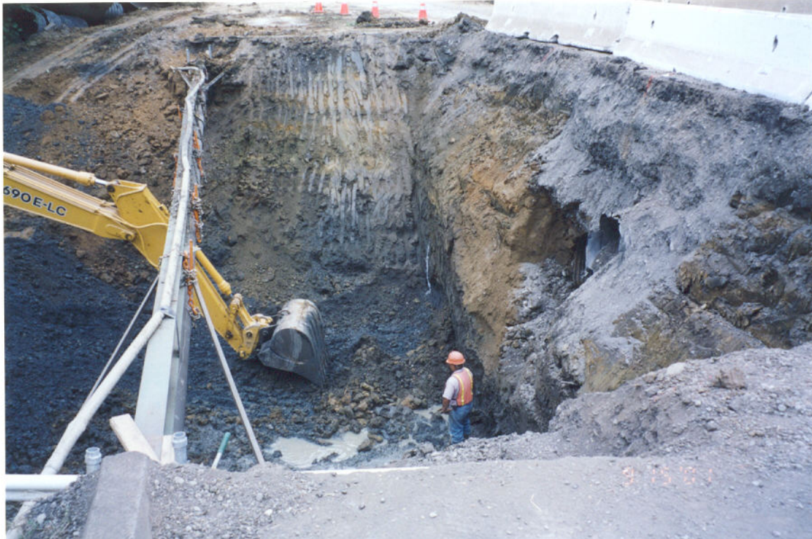
Excavation Prior to Placement of Temporary Flatcar Bridge
