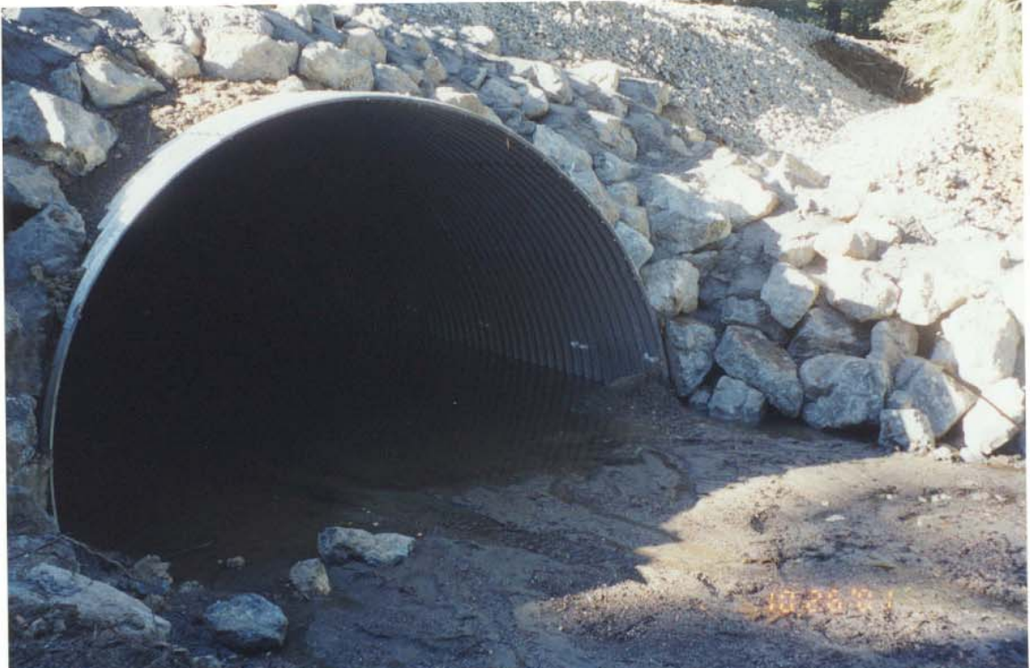
Inlet Rip Rap before Being Concreted
