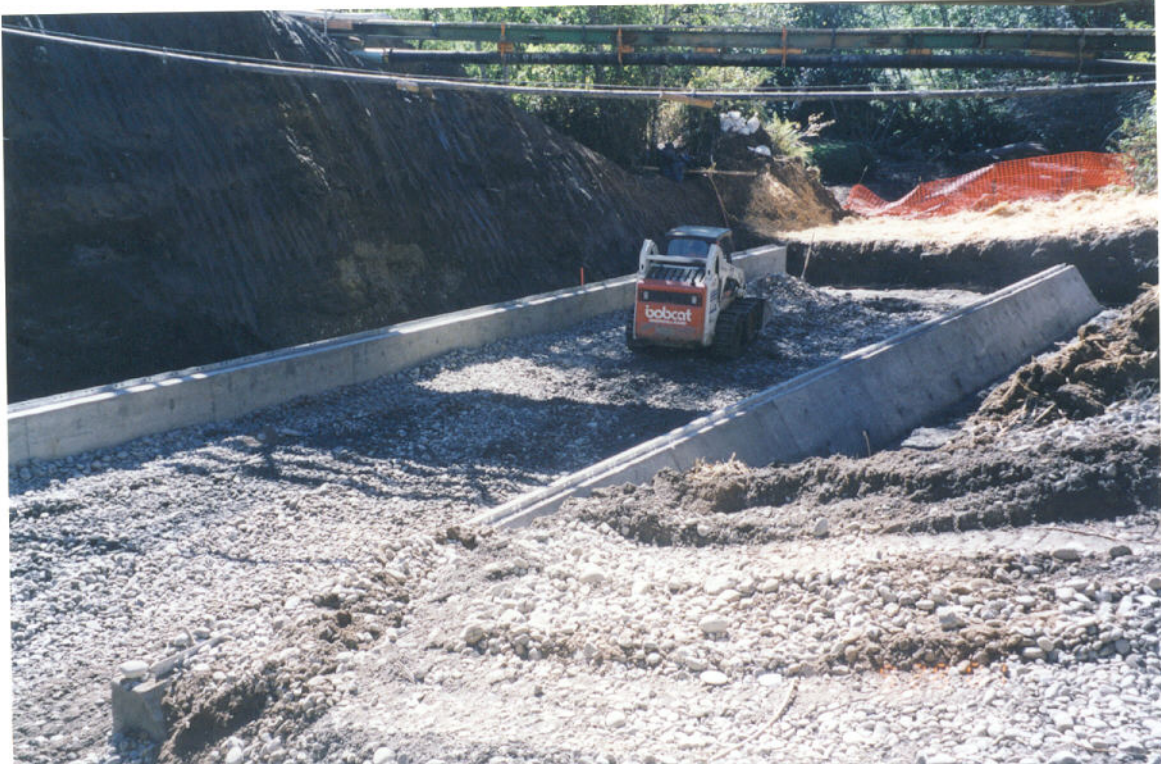
River Gravel Stream Channel Backfill
