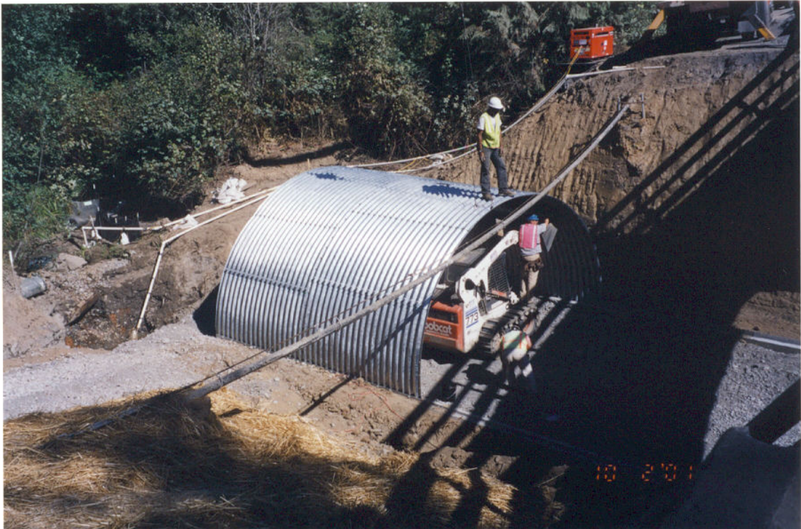
Assembly of Arch Panels
