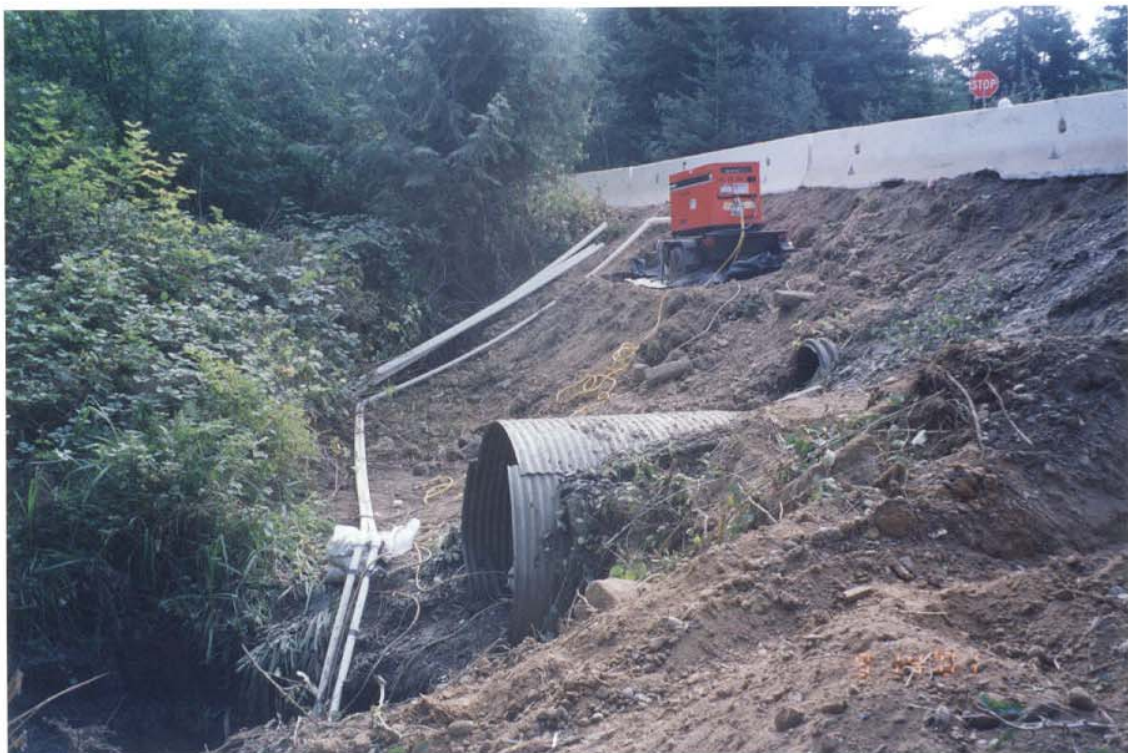
Creek Flow was Pumped around the Project
