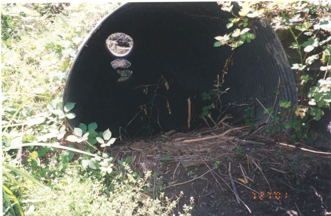
Debris Dam in inlet and Deteriorated Condition of Culvert
