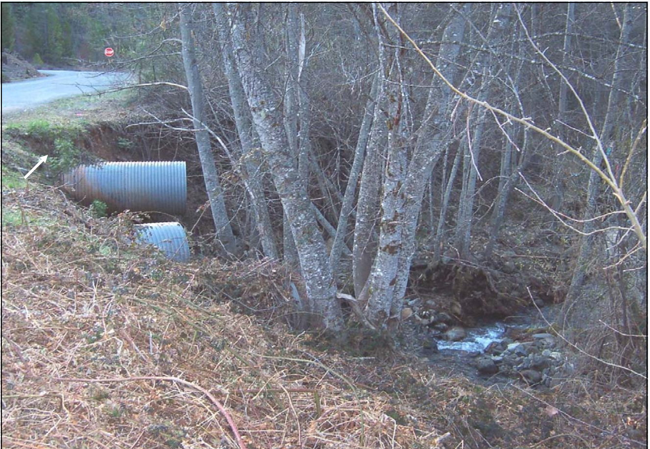
Top : Upstream of the 3, 48" Culverts ~1,400 cyds of Aggraded Sediment Resulted in a Flat, Widened Stream Channel Condition for ~200 Feet Bottom : View of the 3 Perched Outlets & Progressing Outboard Fill Failure
