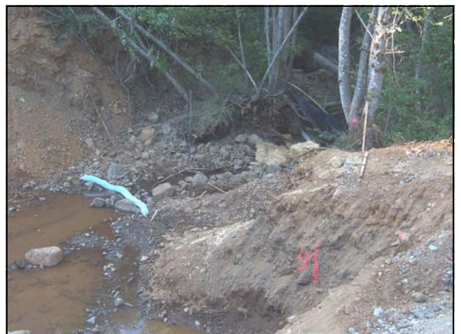
Bottom Right: Straw Bales, Silt Fence & Oil Absorbing Boom Installed below Project
