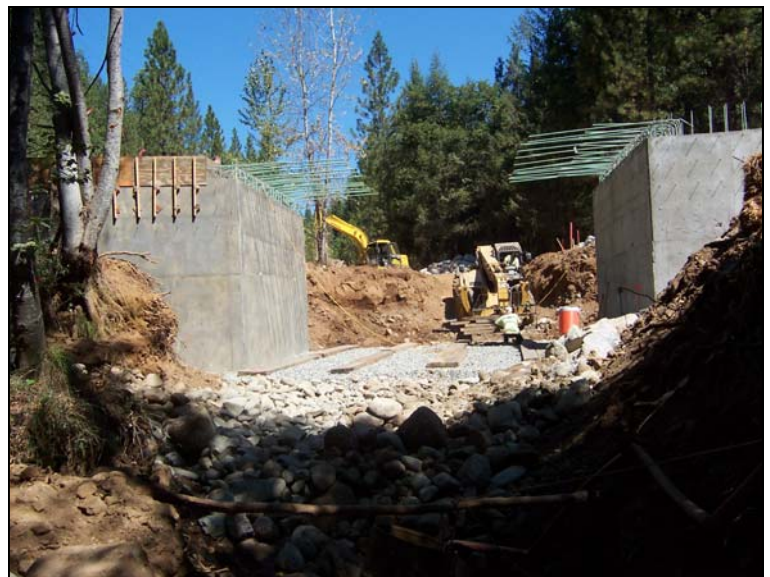
Bottom Right: Abutments Placed & Forms Removed
