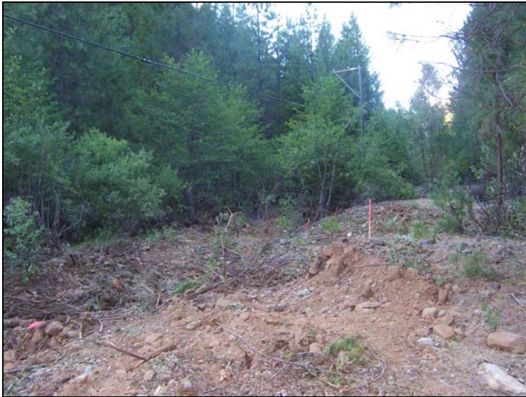
Left: Upstream Channel Vegetation Clearing for Detour & Roughened Channel Construction
