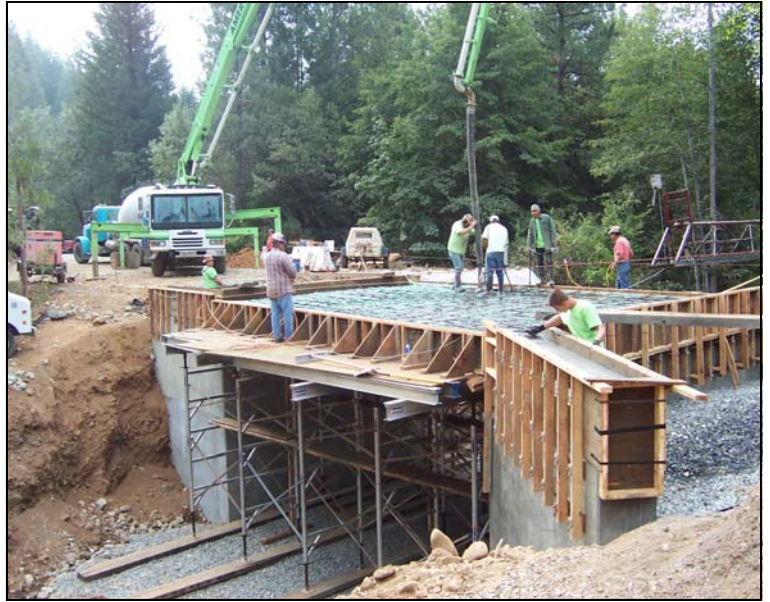
Top Left & Right: Bridge Deck Falsework Construction & Deck Framing/Placing
