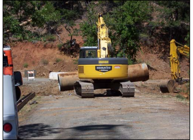
Top: Excavating the 3, 48” Culverts from Roundy Road
