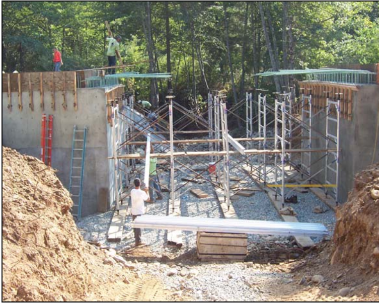
Top Left & Right: Bridge Deck Falsework Construction & Deck Framing/Placing
