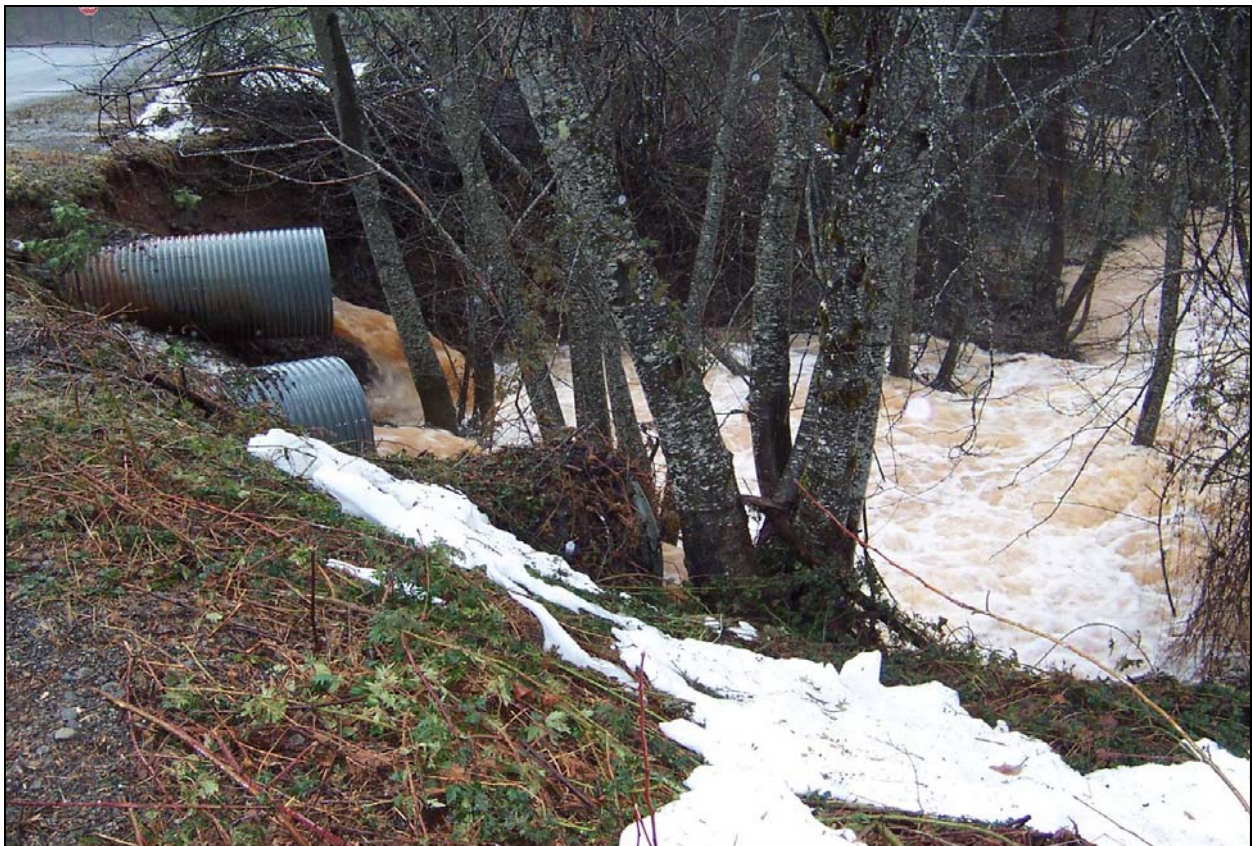
Top : Inlet During High Flow with Submergence & Flooding of Upstream Channel Bottom : Outlet During High Flows
