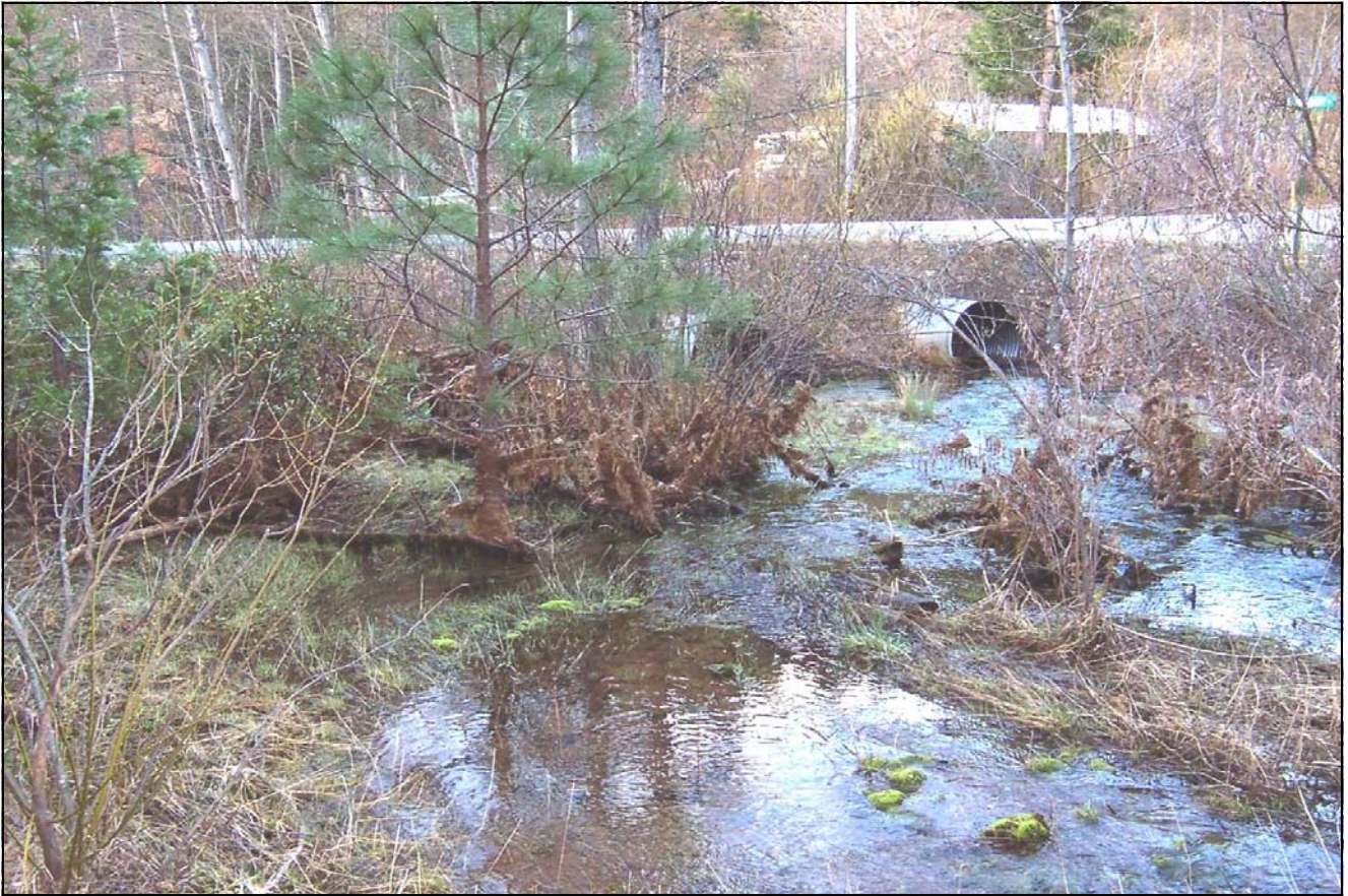
Top : Upstream of the 3, 48" Culverts ~1,400 cyds of Aggraded Sediment Resulted in a Flat, Widened Stream Channel Condition for ~200 Feet Bottom : View of the 3 Perched Outlets & Progressing Outboard Fill Failure
