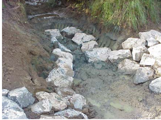
Figure 28 Grade Control Finished
