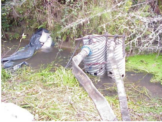
Figure 9 By-Pass System Upstream from Culvert
