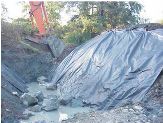
Figure 19 Installing Rip Rap Rock
