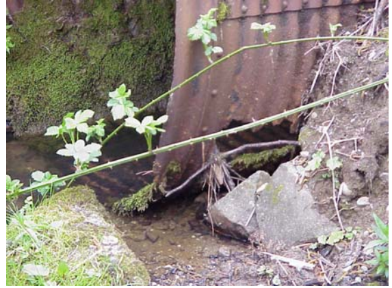
Figure 4 Deteriorated Corrugated Metal Pipe
