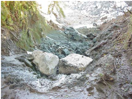
Figure 23 Installing Upstream Grade Control
