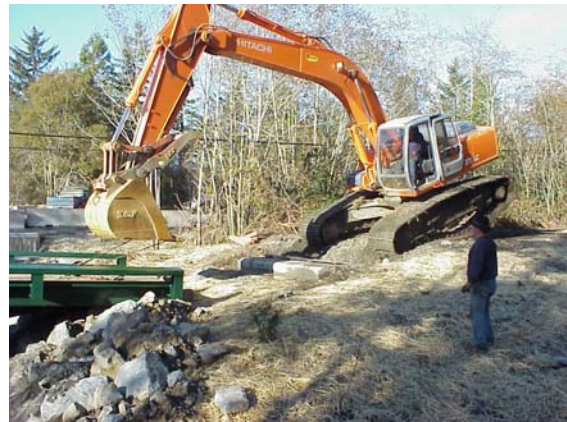
Figure 48 Excavator Lifting Bridge in Place
