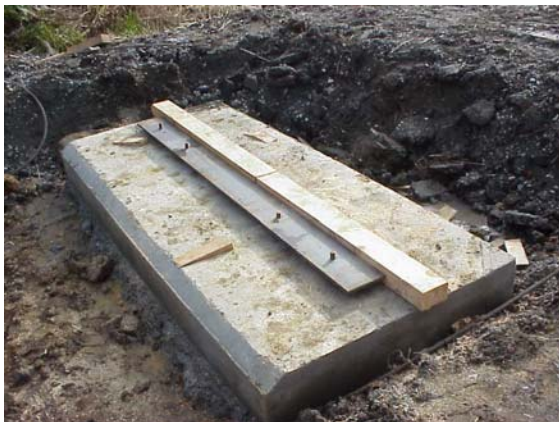
Figure 43 Preparing the Concrete Footing for Flatcar Bridge
