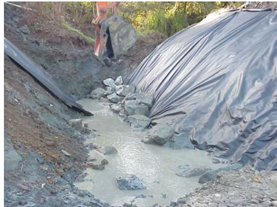
Figure 20 Installing Rip Rap Rock
