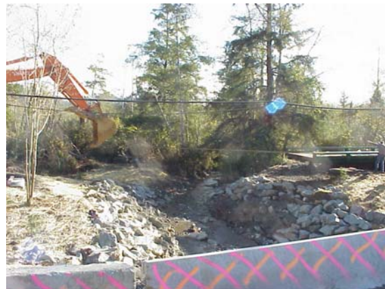
Figure 44 Pulling Flatcar Bridge over the Creek
