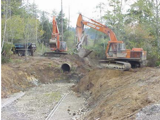
Figure 15 Removal of Twin Culverts
