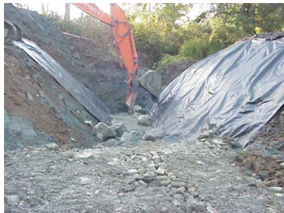
Figure 18 Installing Rip Rap Rock
