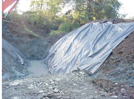
Figure 16 Reconstructing Stream Channel
