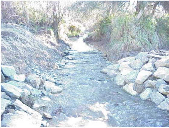
Figure 51 Grade Control After Several Months of Flow
