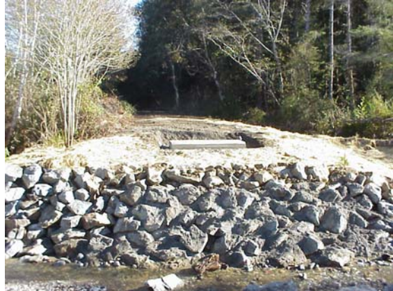
Figure 34 Concrete Footing Placement on Eastbank
