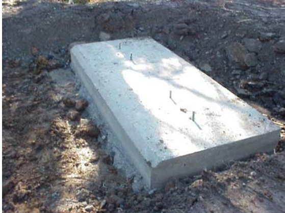
Figure 33 Concrete Footing for Flatcar Bridge
