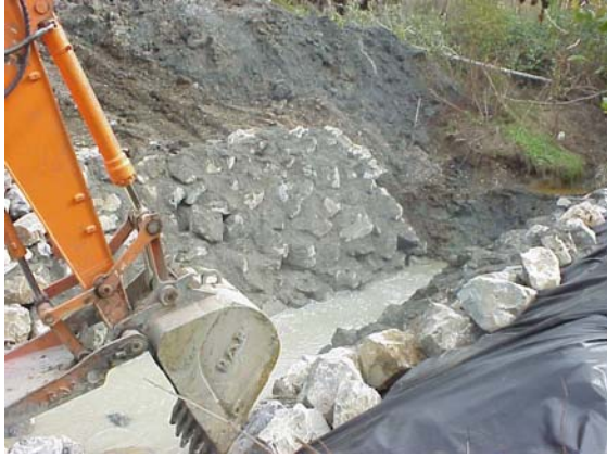
Figure 21 Installing Concreted-Rock Slope Protection
