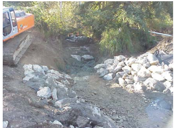
Figure 24 Installing Upstream Grade Control
