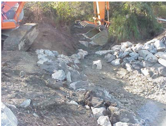
Figure 25 Installing Upstream Grade Control
