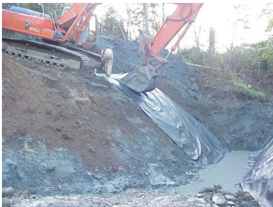
Figure 17 Reconstructing Streambanks
