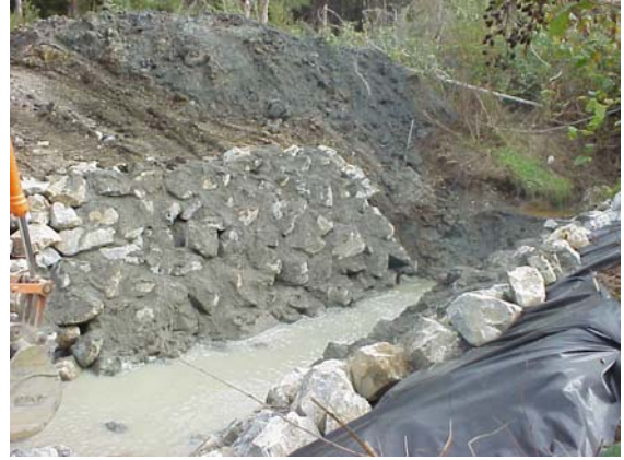
Figure 22 Finished Concrete-RSP
