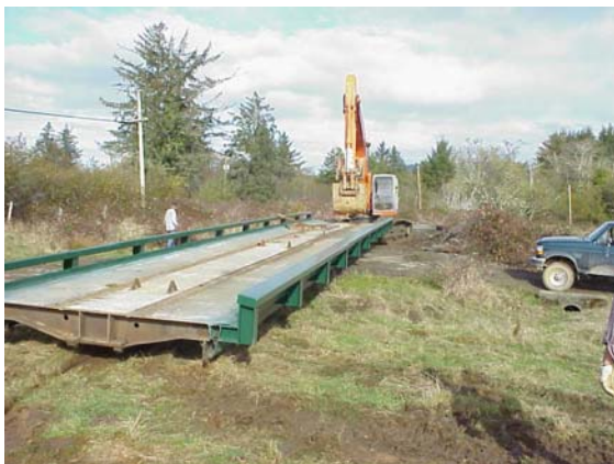
Figure 41 Dragging Flatcar Bridge to Project Site
