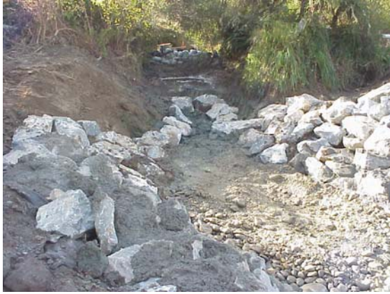
Figure 27 Grade Control Finished
