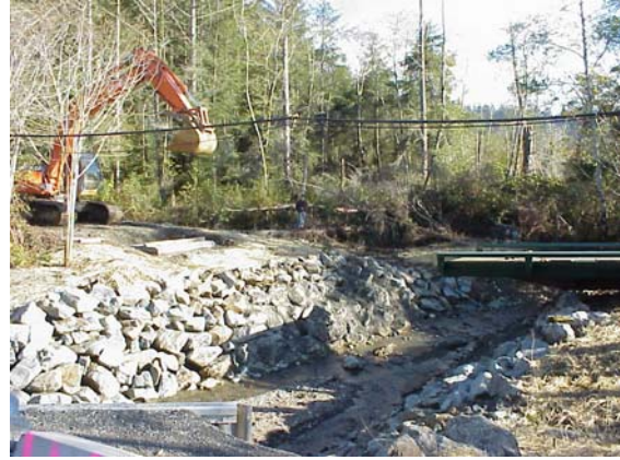
Figure 46 Flatcar Bridge Halfway Across Creek
