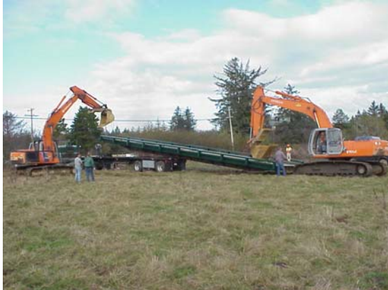
Figure 39 Unloading Flatcar Bridge from Trailer
