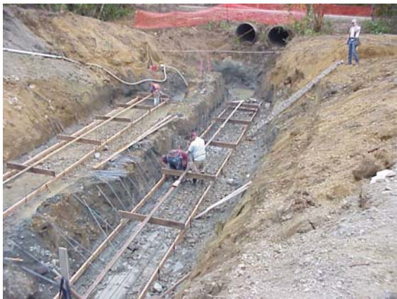
Figure 13 New Footings for Upstream Structure
