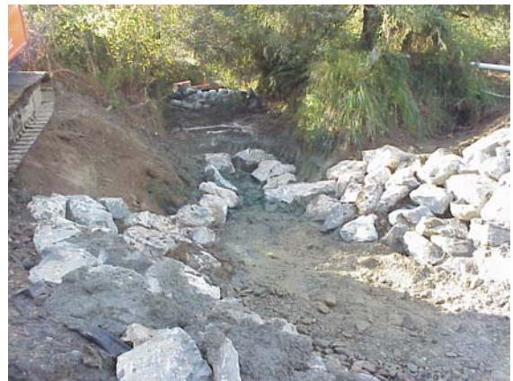
Figure 26 Grade Control Finished
