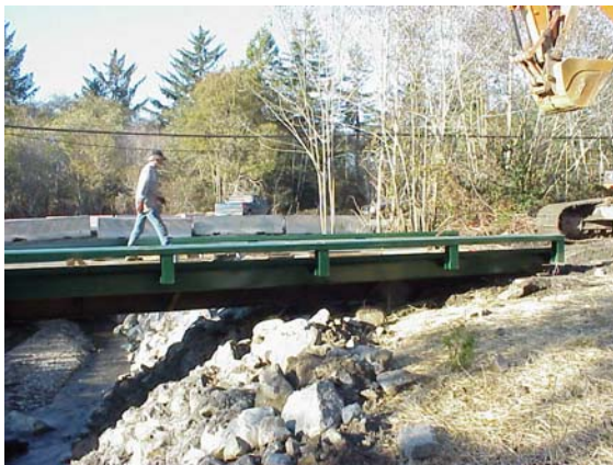
Figure 49 Flatcar Bridge in Final Position Eastbank
