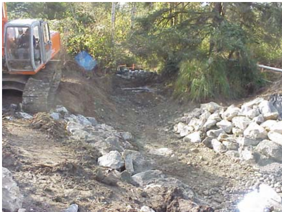
Figure 29 Covering Grade Control with River Run
