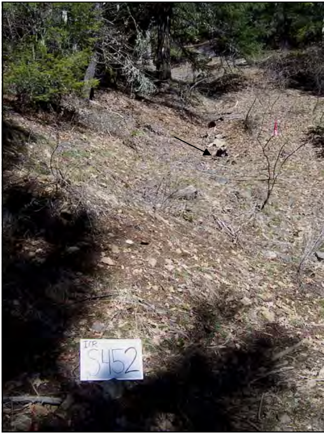
Site 452—Milepost 6.74—Treated Erosion: ~110 cyds Class 3 fill crossing ~155' down right of the bridge over Indian Creek near Cannon Ball Flat. Stream parallel to an old road bed. Treatment: Install rolling dip ~67 feet down left of the crossing Top photos are of crossing channel (black arrow) & the County Road prior to implementation Bottom photo is the installed rolling dip with a rocked overside drain on the left—photo board is on the crest of the dip
