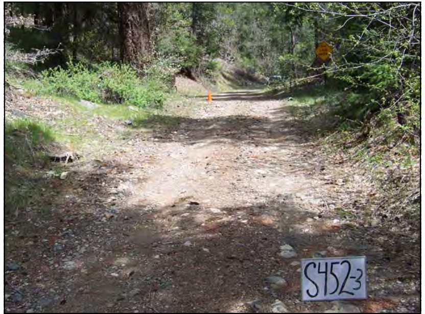
Site 452—Milepost 6.74—Treated Erosion: ~110 cyds Class 3 fill crossing ~155' down right of the bridge over Indian Creek near Cannon Ball Flat. Stream parallel to an old road bed. Treatment: Install rolling dip ~67 feet down left of the crossing Top photos are of crossing channel (black arrow) & the County Road prior to implementation Bottom photo is the installed rolling dip with a rocked overside drain on the left—photo board is on the crest of the dip
