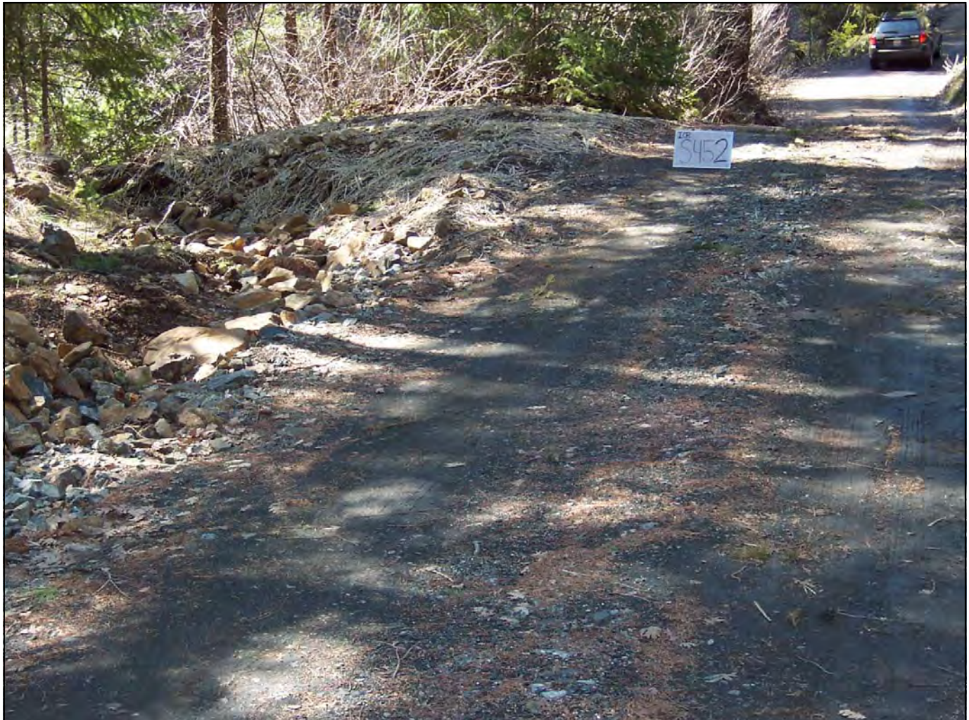
Site 452—Milepost 6.74—Treated Erosion: ~110 cyds Class 3 fill crossing ~155' down right of the bridge over Indian Creek near Cannon Ball Flat. Stream parallel to an old road bed. Treatment: Install rolling dip ~67 feet down left of the crossing Top photos are of crossing channel (black arrow) & the County Road prior to implementation Bottom photo is the installed rolling dip with a rocked overside drain on the left—photo board is on the crest of the dip
