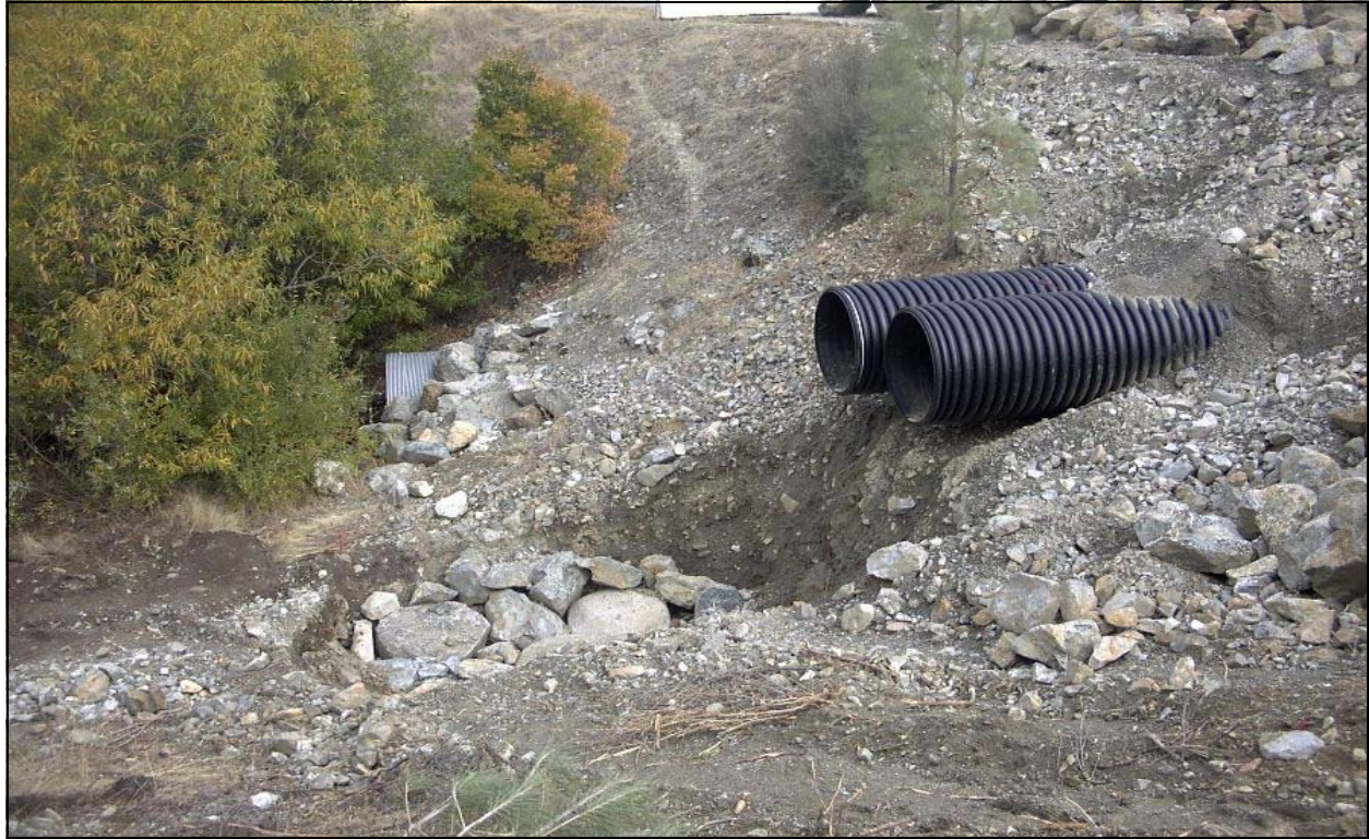
Above: Side view of overflow culvert outlets without rock slope protection (Phase 2)
