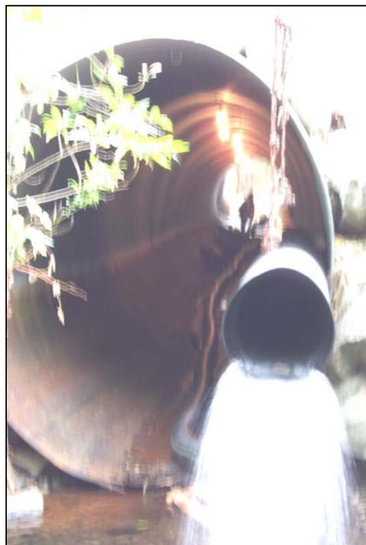
Utilizing a stud gun to weld bolts to the inner walls of the culvert in order to suspend the diversion pipe and hang lighting and cordage from above (Phase 3)
