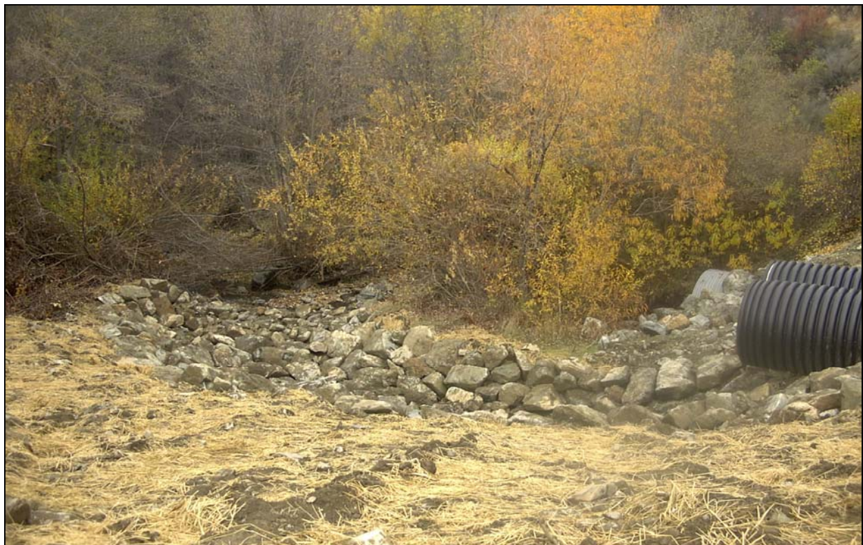
Below: Same view of overflow culvert outlets with rock slope protection and revegetation
