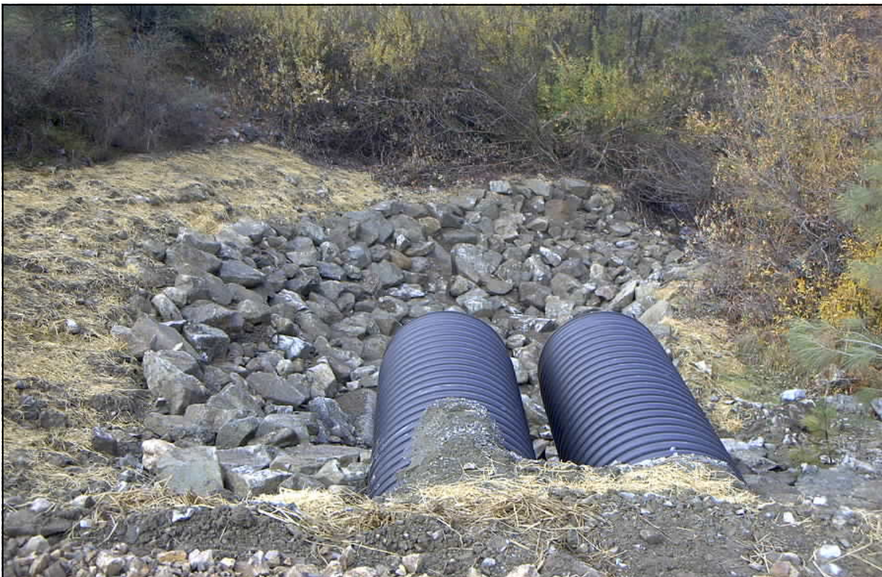
Below: Outlet fillslope of 4-foot diameter HDPE overflow culverts with RSP
