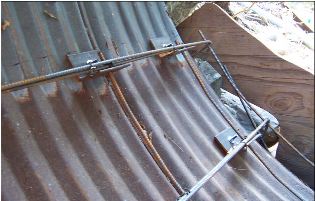
Above & Below: Rebar and baffles set, welded and tied within the culvert bottom. At the Inlet and Outlet, rebar was wrapped on to the outside edges of the culvert and concrete was poured over these edges to create a tight seal (note frame board below)
