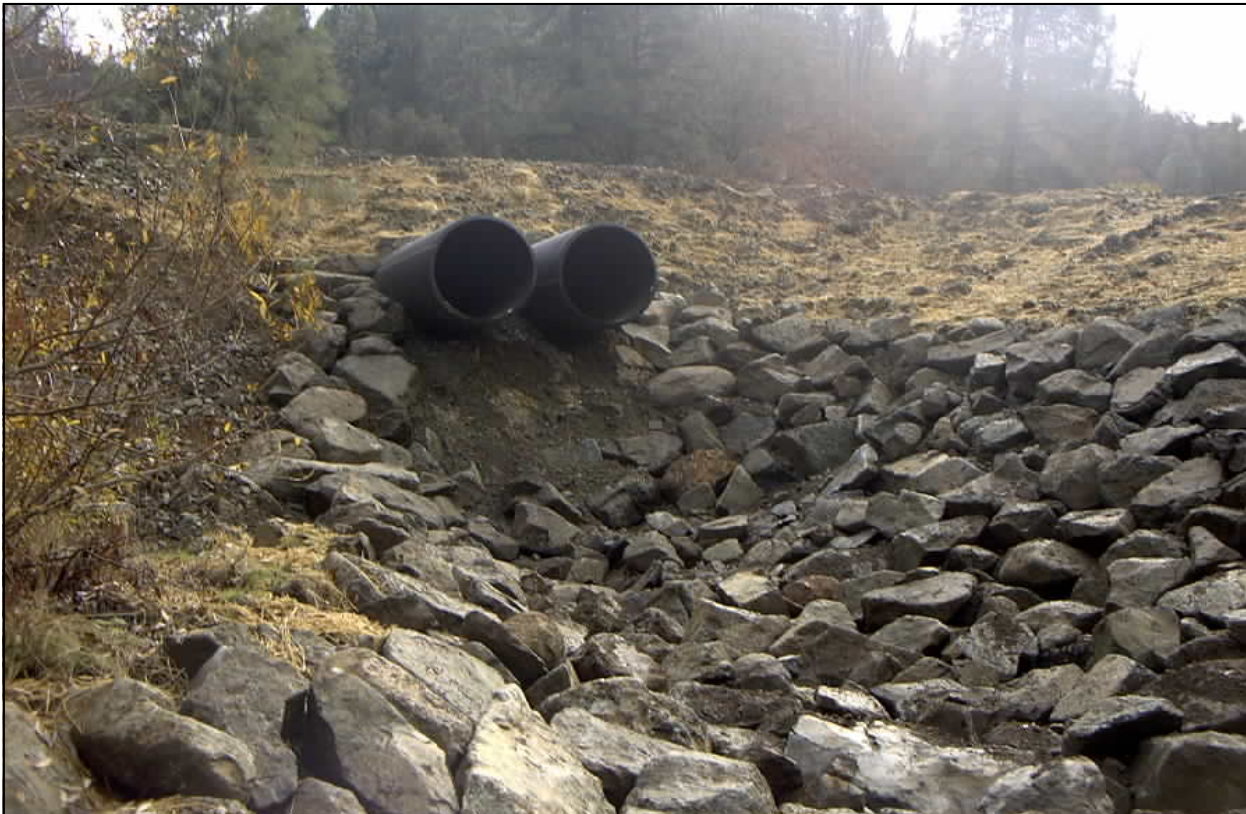
Below: View of overflow pipes and rock slope protection (Phase 2)
