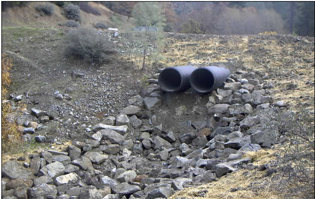
Below: Rock slope protection placed at the overflow culvert outlets
