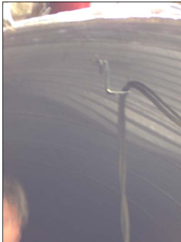
Utilizing a stud gun to weld bolts to the inner walls of the culvert in order to suspend the diversion pipe and hang lighting and cordage from above (Phase 3)
