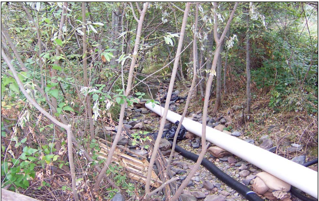
Below: Diversion pipes extending from cofferdam to culvert inlet
