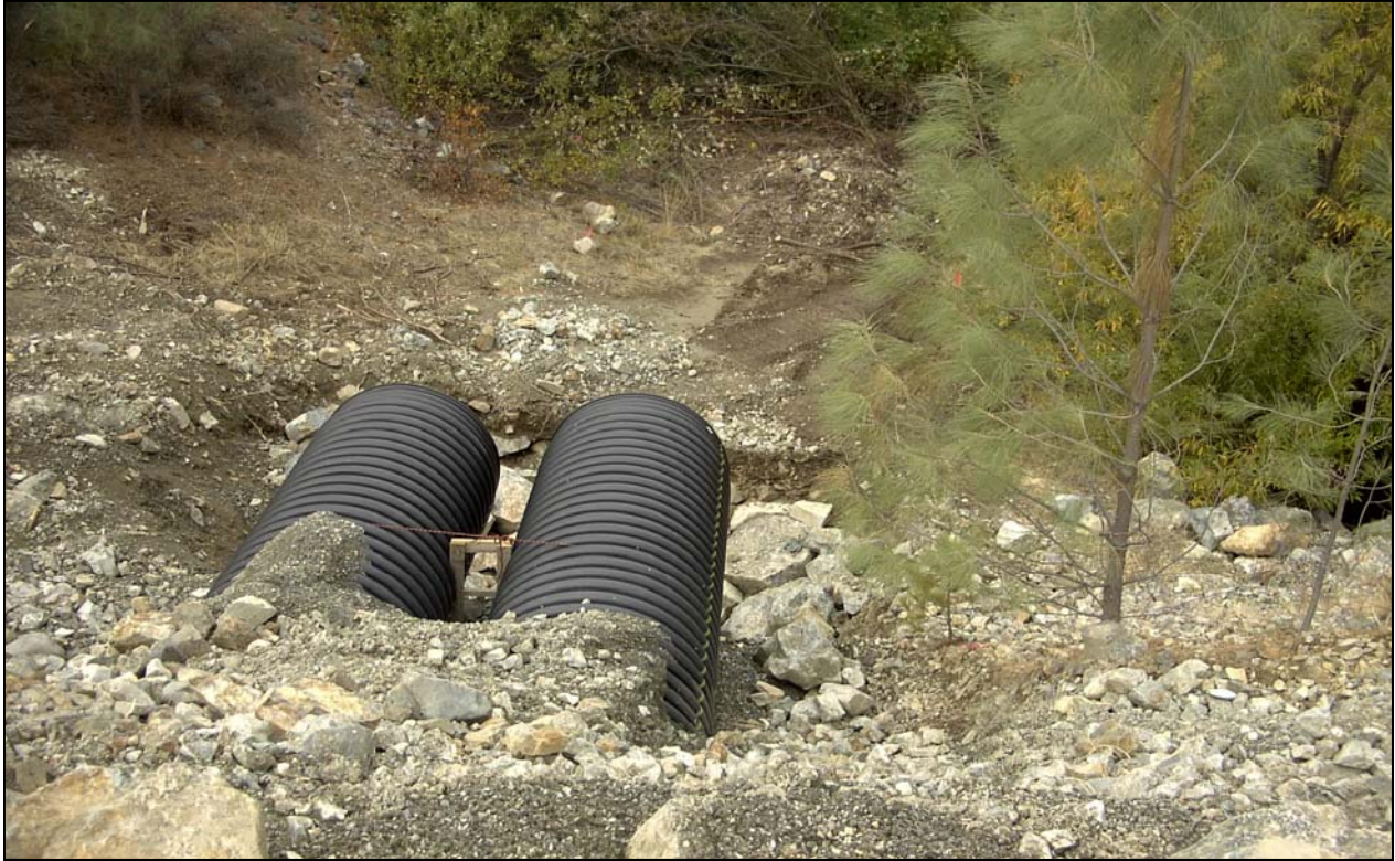
Above: Outlet fillslope of 4-foot diameter HDPE overflow culverts without rock slope Protection (Phase 2)
