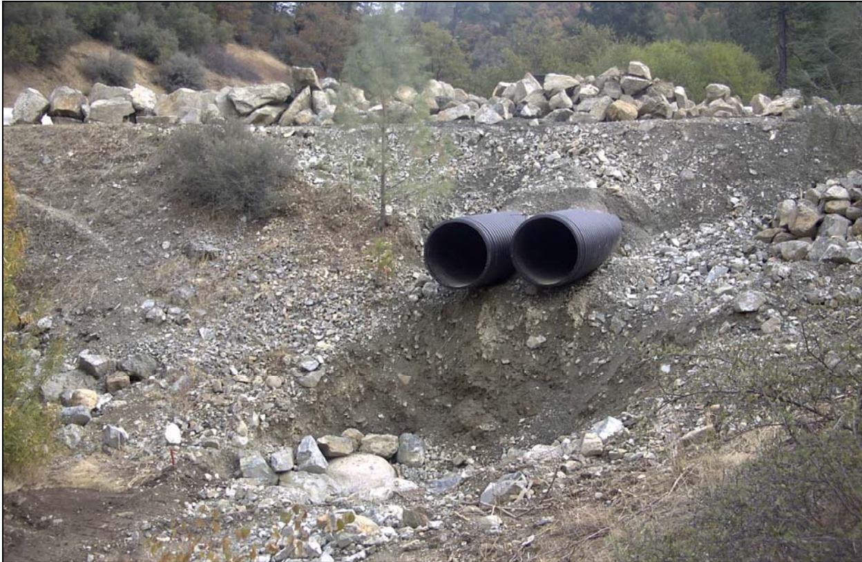
Above: 4-foot diameter overflow culverts installed (rock slope protection is on the road awaiting placement—Phase 2)
