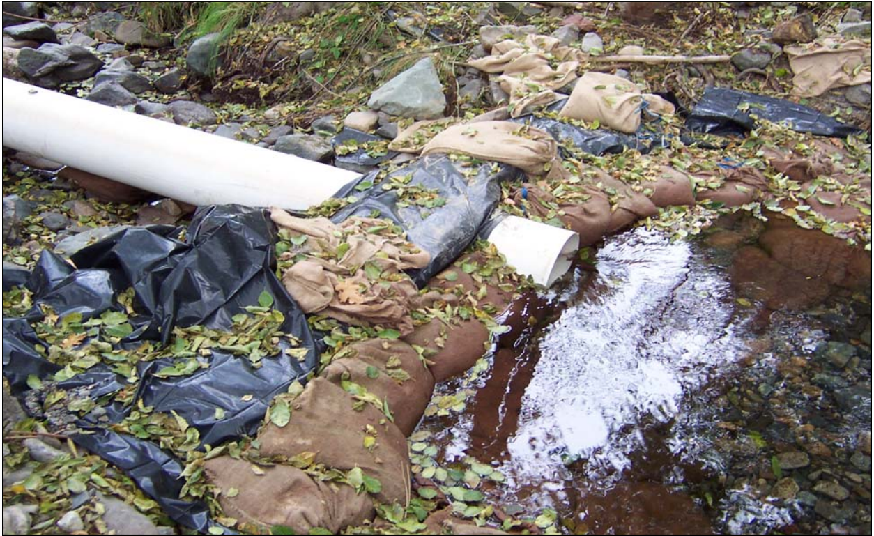
Above: Cofferdam & 15"-inch diversion pipe set approximately 40-feet upstream of the culvert inlet
