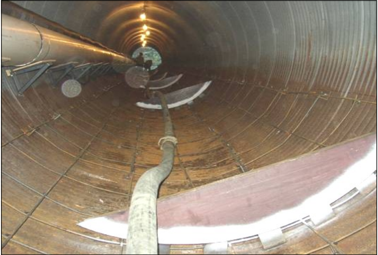
Above & Below: Rebar and baffles set, welded and tied within the culvert bottom. At the Inlet and Outlet, rebar was wrapped on to the outside edges of the culvert and concrete was poured over these edges to create a tight seal (note frame board below)
