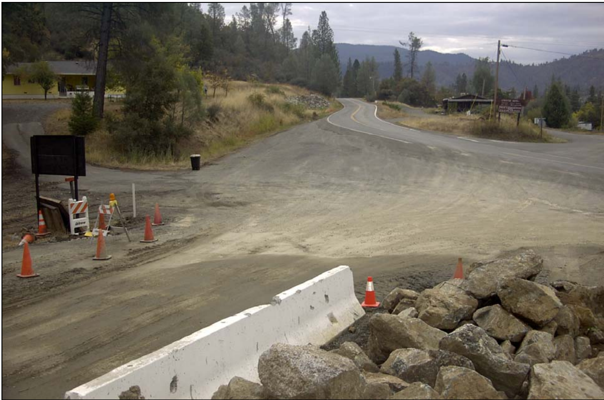
Above: Rock Slope protection and road surface prior to placement and resurfacing
