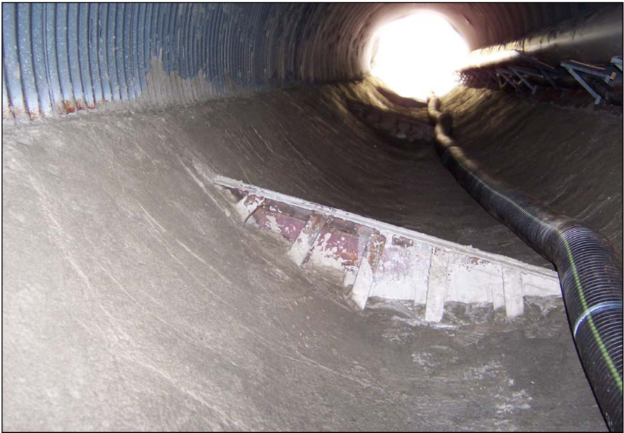
Above: One baffle set in the concrete—view looking upstream from culvert outlet
