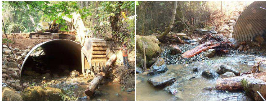
Installing large wood at the culvert outlet (left) and completed LWD (right)
