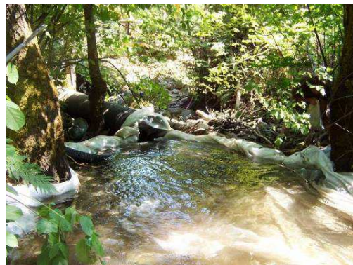
Left: The initial water diversion pipe placed within the old culvert was used to allow excavation of the road fill and installation of the main diversion pipe, which is visible in the right side of the photo. Once the main diversion pipe was installed, the initial diversion pipe in the 10' diameter CMP was removed. Right: Diversion Dam upstream of the project
