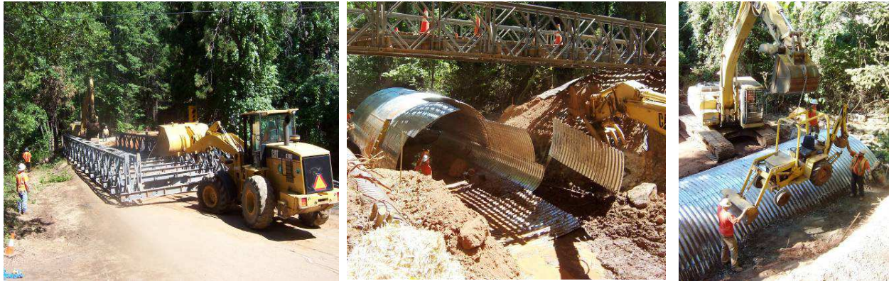
Half width construction was possible with the use of a bailey bridge. Left: Bailey bridge installation, Middle: construction of the multiplate in place, underneath the bridge, Right: lowering the small backhoe into place alongside the newly constructed pipe.
