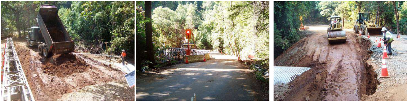
Constructing the upstream fill material (left), the detour road and traffic control lights (middle), constructing the downstream fill (right).
