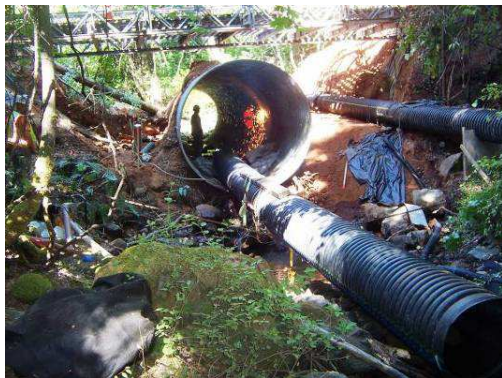
Left: The initial water diversion pipe placed within the old culvert was used to allow excavation of the road fill and installation of the main diversion pipe, which is visible in the right side of the photo. Once the main diversion pipe was installed, the initial diversion pipe in the 10' diameter CMP was removed. Right: Diversion Dam upstream of the project
