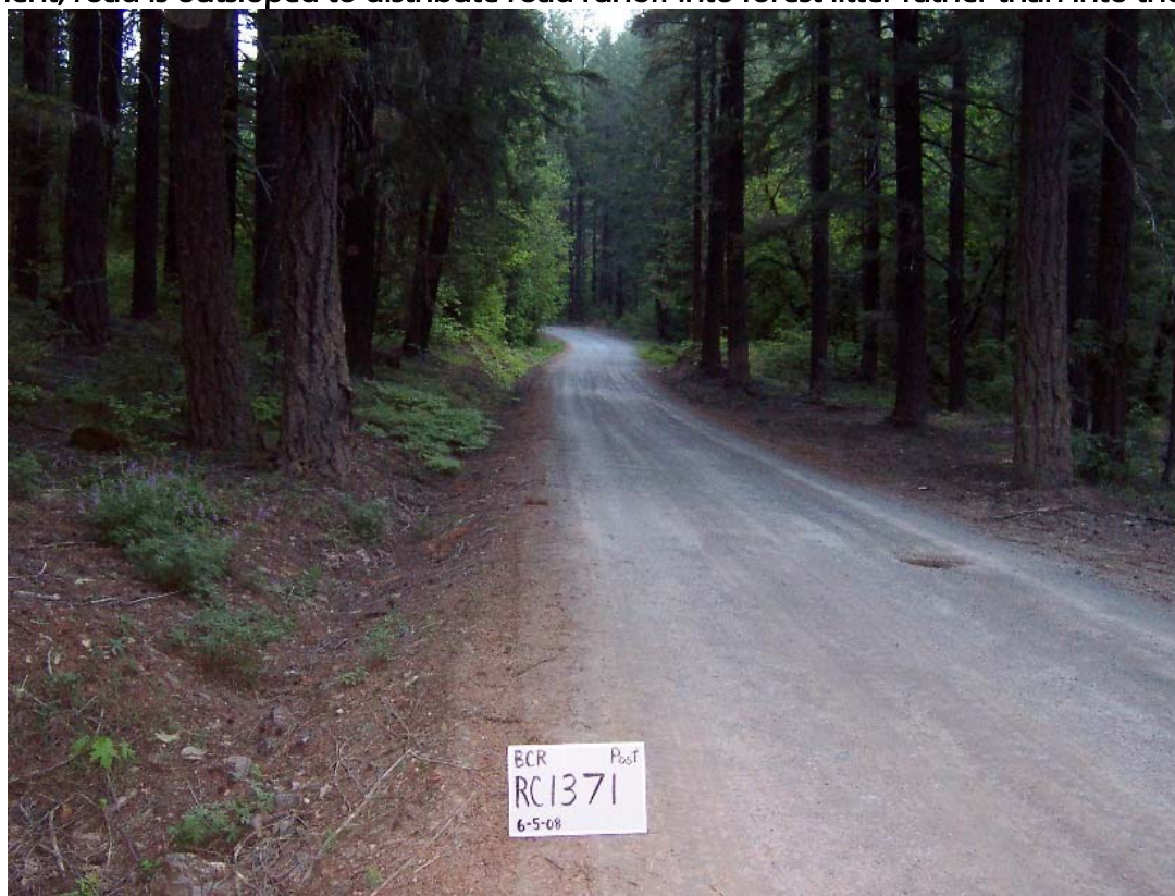
Photo1 (above). Site 1371 Showing in-sloped road draining to ditch and culvert. Photo 2 (below). Post treatment, road is outsloped to distribute road runoff into forest litter rather than into the ditch.
