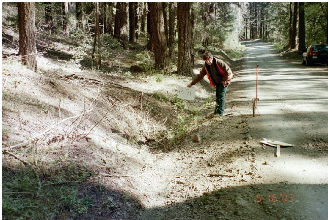
Photo1 (above). Site 1371 Showing in-sloped road draining to ditch and culvert. Photo 2 (below). Post treatment, road is outsloped to distribute road runoff into forest litter rather than into the ditch.
