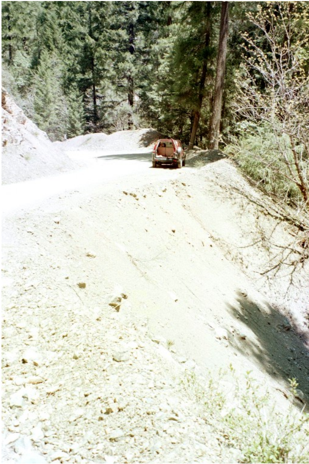
Photo 13 (above left). An extremely narrow road segment with a large berm and spoils area near Big Creek (Site 1383). Photo 14 (above right) shows the spoils removed. Photo 14 also shows the road improvement and widening which was done as a separate project.
