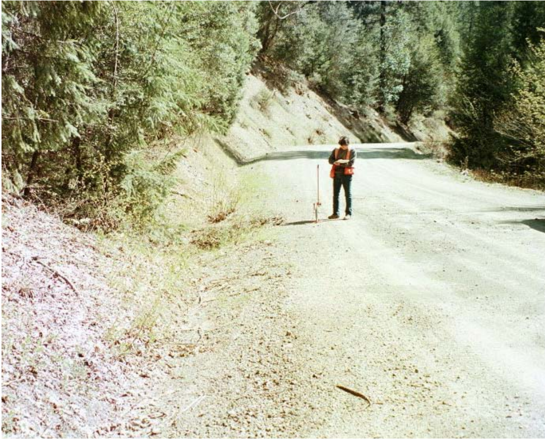
Photo 3 (above). Site 1374 (before project), showing segment of in-sloped road that was outsloped with retention of the ditch segment (Photo 4, below).
