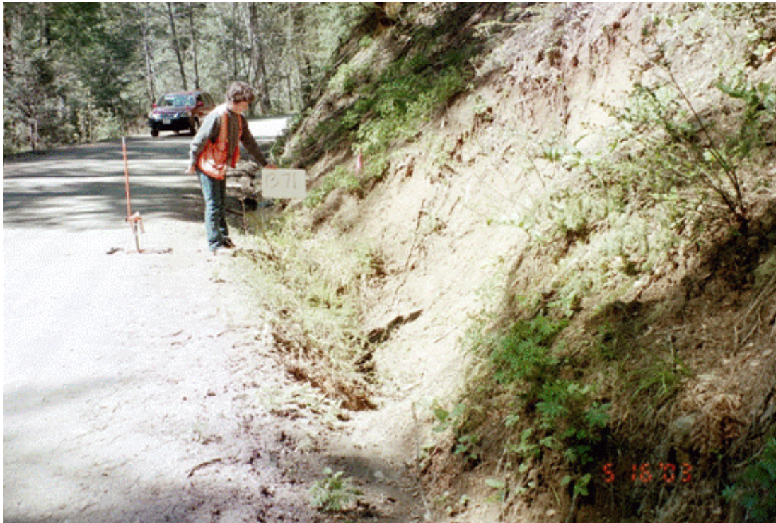
Photo 5 (above). Site 1376 consisted of 880' of ditch system delivering from both directions to an 18" ditch relief culvert (above). This culvert had a "shot gun" outlet. Photo 6 (below). The site treatment included installation of a drop inlet on the culvert to prevent plugging from cutbank sluff, outsloping the road, cutting the shot gun culvert and installing rock armor outlet.
