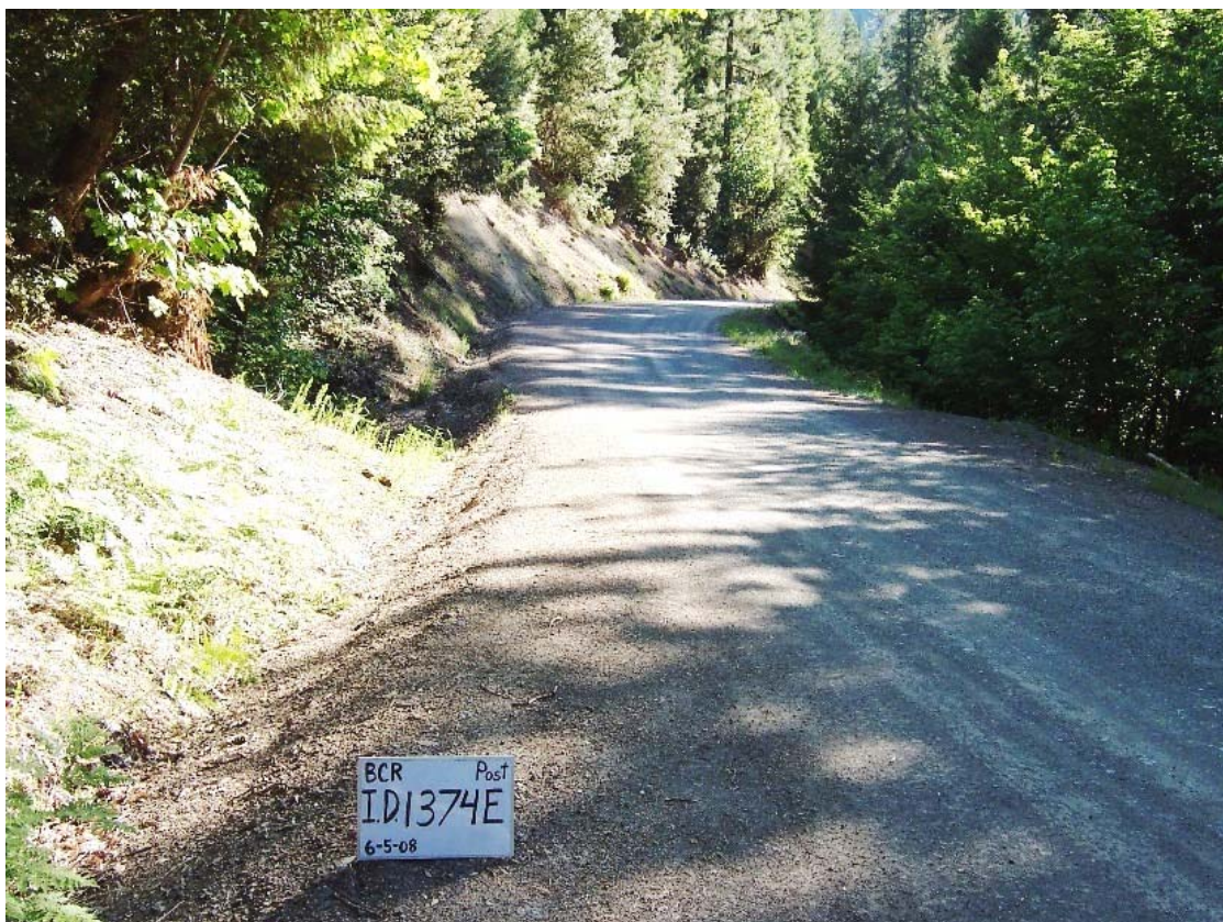
Photo 3 (above). Site 1374 (before project), showing segment of in-sloped road that was outsloped with retention of the ditch segment (Photo 4, below).
