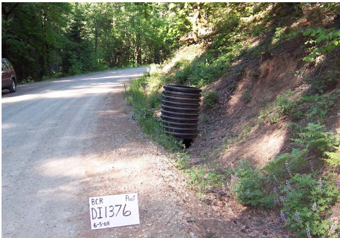
Photo 5 (above). Site 1376 consisted of 880' of ditch system delivering from both directions to an 18" ditch relief culvert (above). This culvert had a "shot gun" outlet. Photo 6 (below). The site treatment included installation of a drop inlet on the culvert to prevent plugging from cutbank sluff, outsloping the road, cutting the shot gun culvert and installing rock armor outlet.
