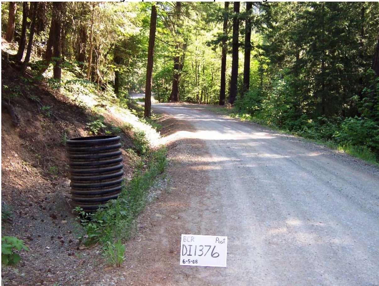
Photo 7 (above). Site 1376. Looking from the other side of the ditch from Photo 5, Photo 8 (below) showing drop inlet and outsloped road segment.
