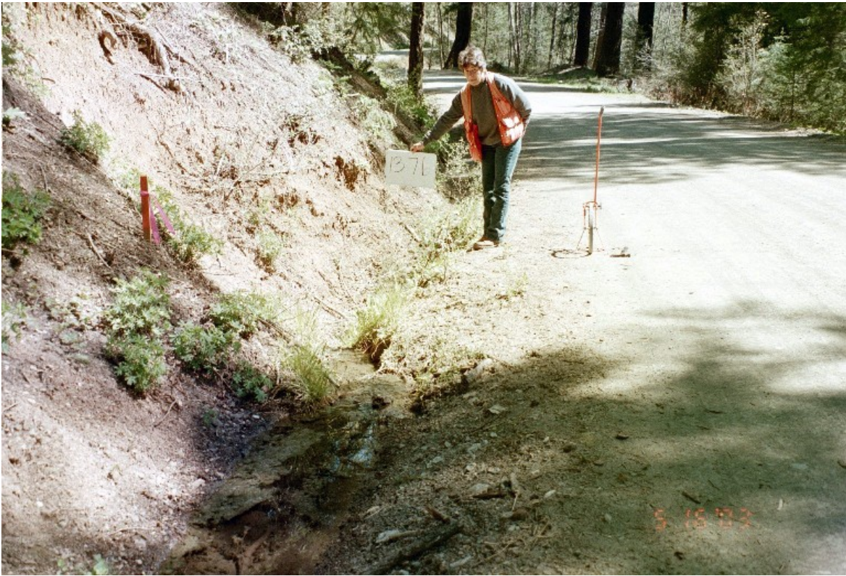
Photo 7 (above). Site 1376. Looking from the other side of the ditch from Photo 5, Photo 8 (below) showing drop inlet and outsloped road segment.
