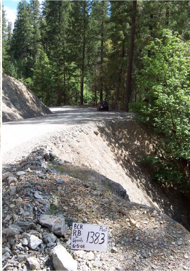
Photo 13 (above left). An extremely narrow road segment with a large berm and spoils area near Big Creek (Site 1383). Photo 14 (above right) shows the spoils removed. Photo 14 also shows the road improvement and widening which was done as a separate project.
