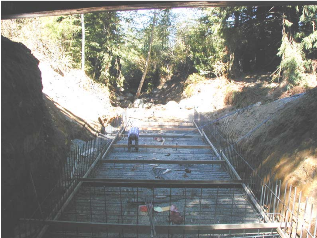
INSTALLING REBAR & FORMS FOR CULVERT BASE
