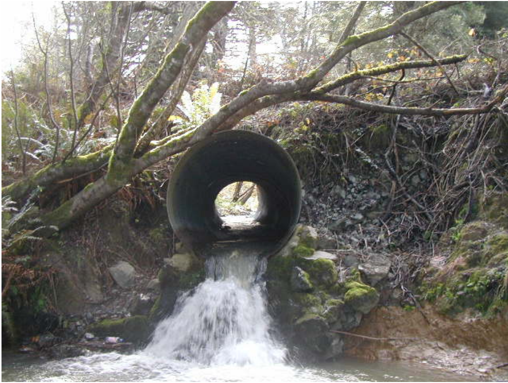
CULVERT OUTLET PRIOR TO CONSTRUCTION
