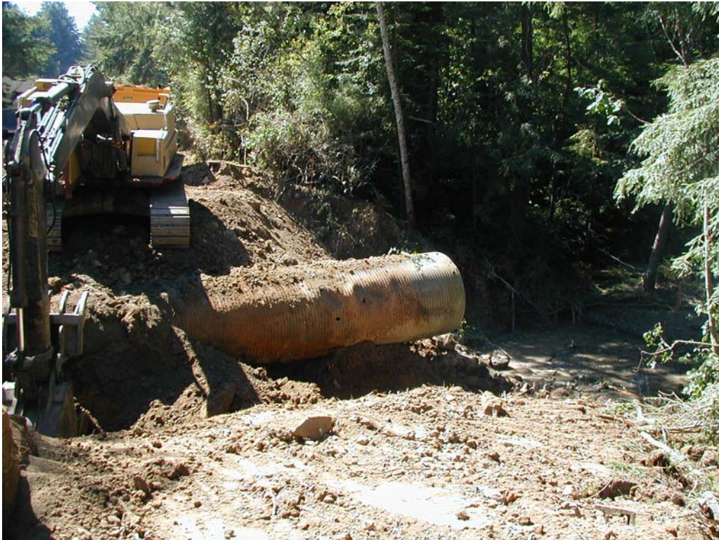
EXCAVATING & REMOVING EXISTING CULVERT
