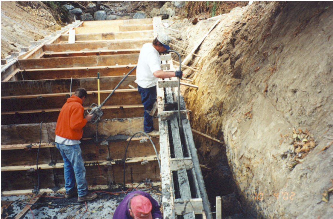
POURING WALLS AND WEIRS
