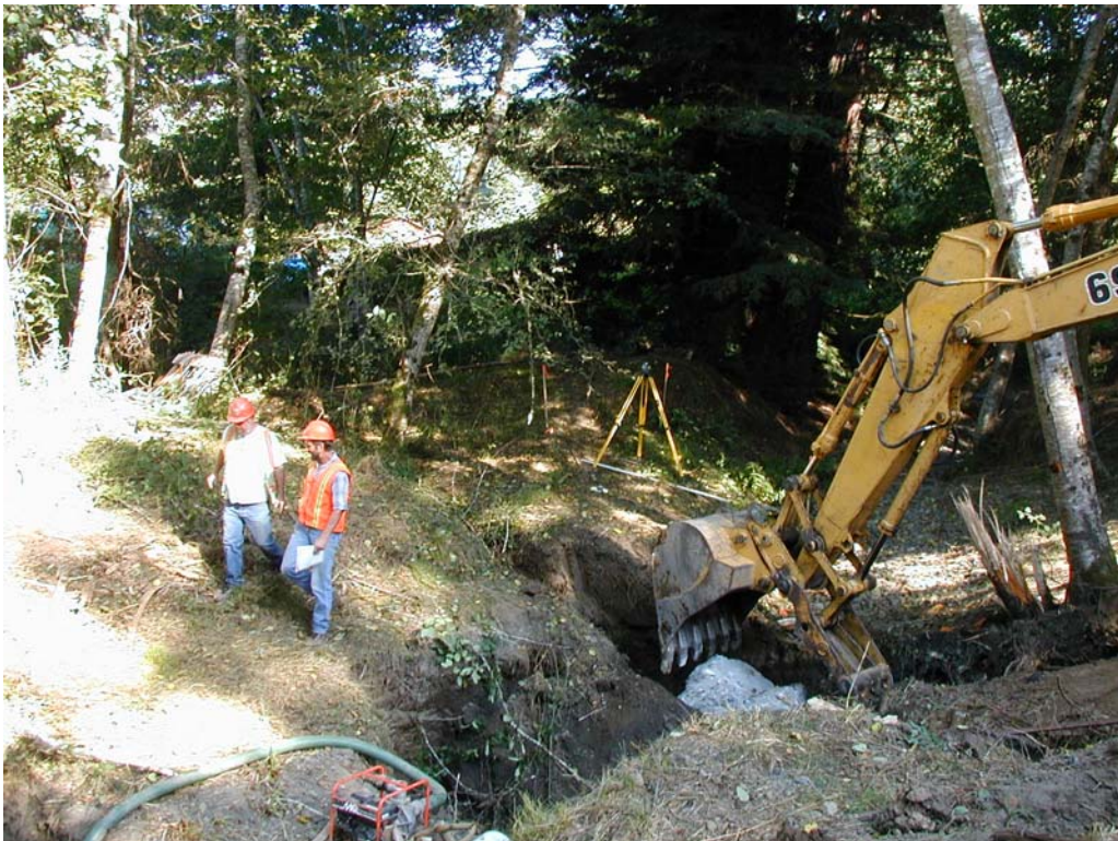
INSTALLING INSTREAM BOULDER WEIRS
