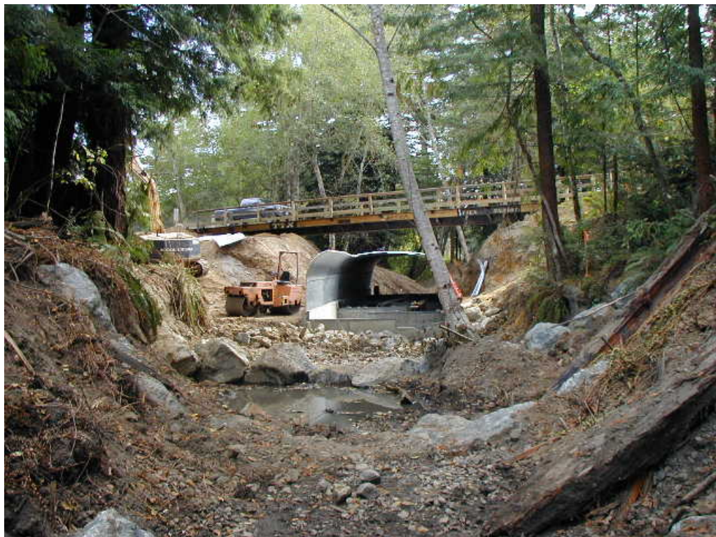
ASSEMBLING CULVERT (VIEW FROM DOWNSTREAM)
