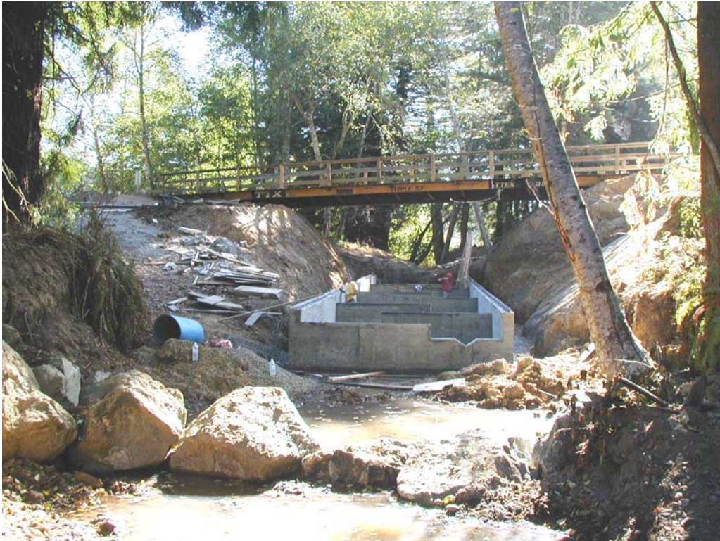
CULVERT BASE COMPLETED (VIEW FROM DOWNSTREAM)
