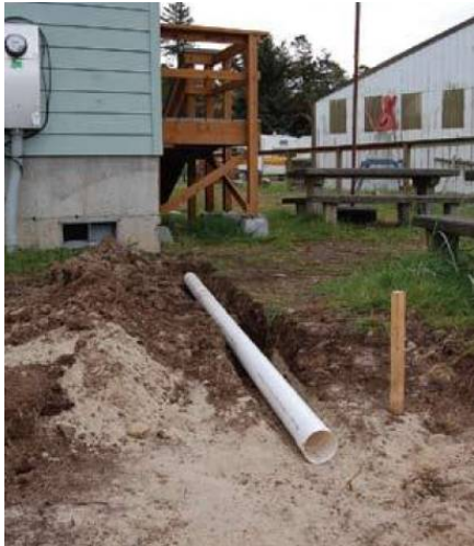
Figure 9 This 4" ABS pipe will convey water from this building into a rain garden. Pipes like these must be laid at a slope dropping about 1 inch for every 10 feet so water flows away from the building but does not build up too much speed by the time it arrives. Per the Plumbing Code, they must be buried at least 12" to the top of the pipe.
