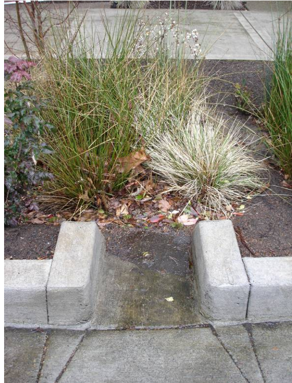
Figure 19 Because of a small amount of sediment and possibly too much vegetation right at the mouth of the inlet, the smallest, most frequent, and dirtiest flows are bypassing the inlet.
