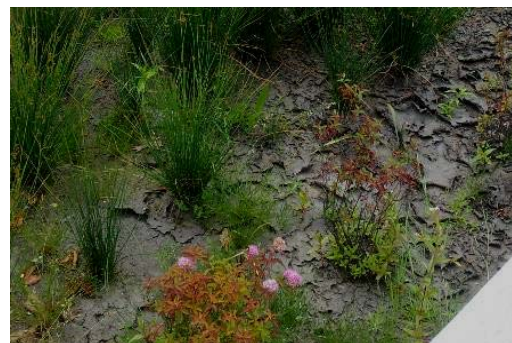
Figure 20 Curled soil often suggests a facility has clogged and ponded water, possibly excessively.
