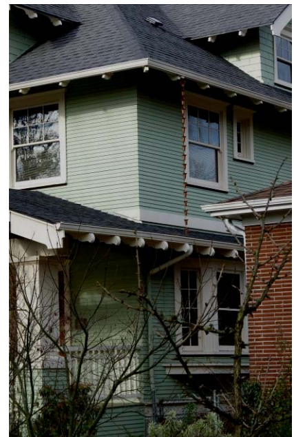
Figure 10 Copper rain chains are a popular, yet polluting, means of slowing water flow. Copper in very small amounts is toxic to fish and other aquatic life. Because it's soluble (can be dissolved) in water, it can't be treated by a rain garden.
