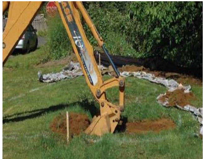
Figure 16 Avoid foot or vehicular traffic before, during, and after construction. This backhoe is excavating from outside the rain garden.
