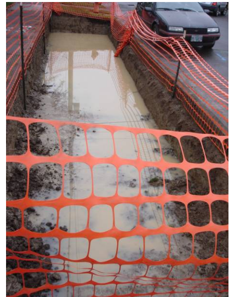
Figure 14 These native soils clogged due to rain exposure and possibly foot traffic during construction. Clayey soils this wet are difficult to unclog since they clump. You probably need to wait for it to evaporate before amending. If left like this, the facility won't infiltrate and plants are likely to die from poor drainage.
