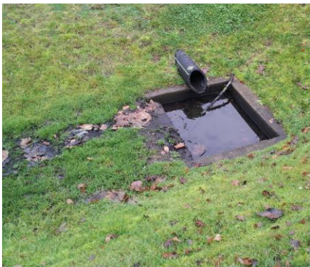
Figure 8 This sump settles sediment from roofs and pavement and makes it easy to remove.
