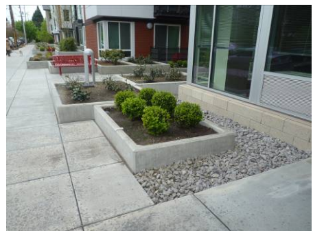
Figure 9 Crushed aggregate can be as aesthetically pleasing as rounded river rock and does a better job at protecting water quality.
