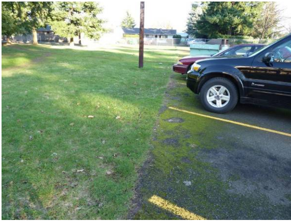
Figure 8 Another accidental vegetated filter strip. The parking lot sheds runoff to the left towards the grassy area. A lack of curbs and additional drainage means all the runoff from the parking lot stays on-site.
