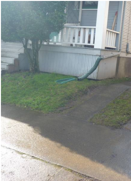
Figure 5 Avoid disconnecting your downspout onto a short hill like this. Instead, attach your downspout to a level spreader (described below) and turn the rest of the yard into a vegetated filter strip.
