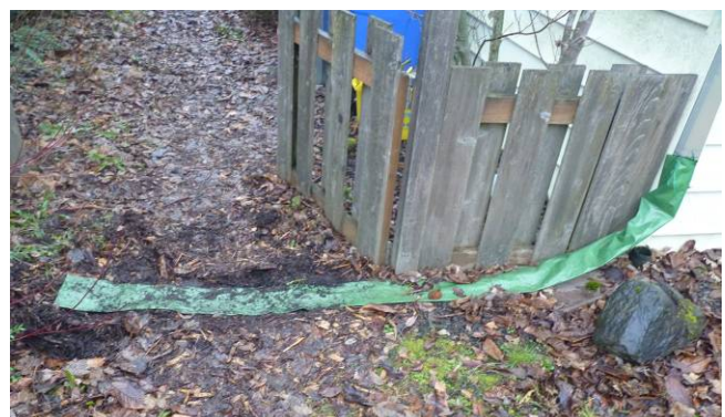
Figure 2 This LDPE downspout extension is next to a slab footing of a garage. A non-perforated section on the right provides adequate setback for a garage slab, while the left half has holes that spread runoff out, preventing erosion. Compost amended soil below and a few inches of mulch added every year to the path surface, make this a no maintenance "facility".
