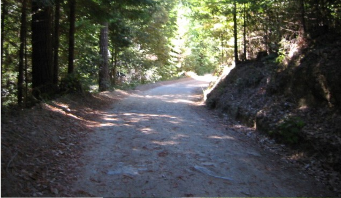
Picture Point 6 AFTER Looking South 30° West After Applying 8" rock and out sloping @ 4%.
