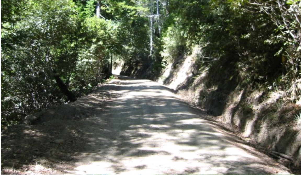
Picture Point 8 AFTER Looking North 40° West After reconfiguring road by Outsloping @ 4% Applying 3" rock. Rolling dip installed at arrow.
