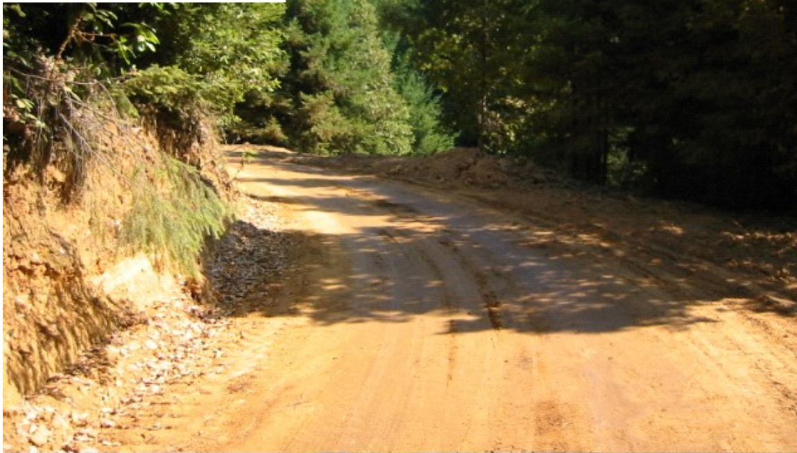
Picture Point 7 AFTER Sep 27, 2002 Mileage: 22.45 to 22.49 Looking East After outslowing @ 4% and applying 8" rock
