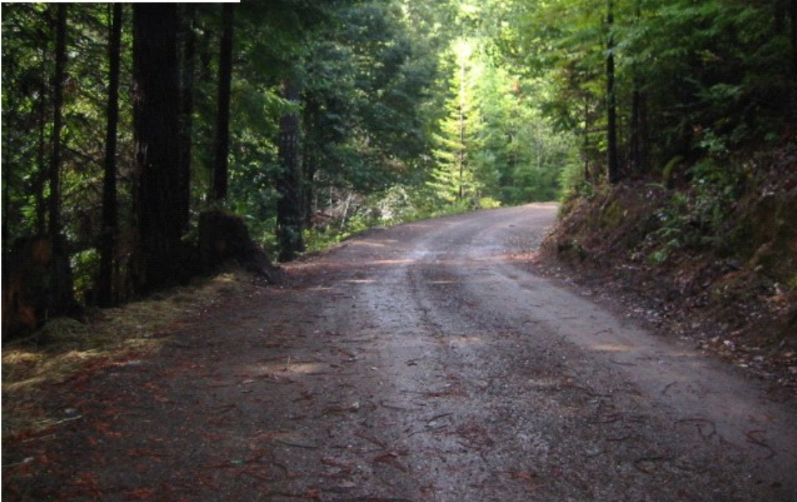
Picture Point 6 AFTER Looking South 30° West After Applying 8" rock and out sloping @ 4%.
